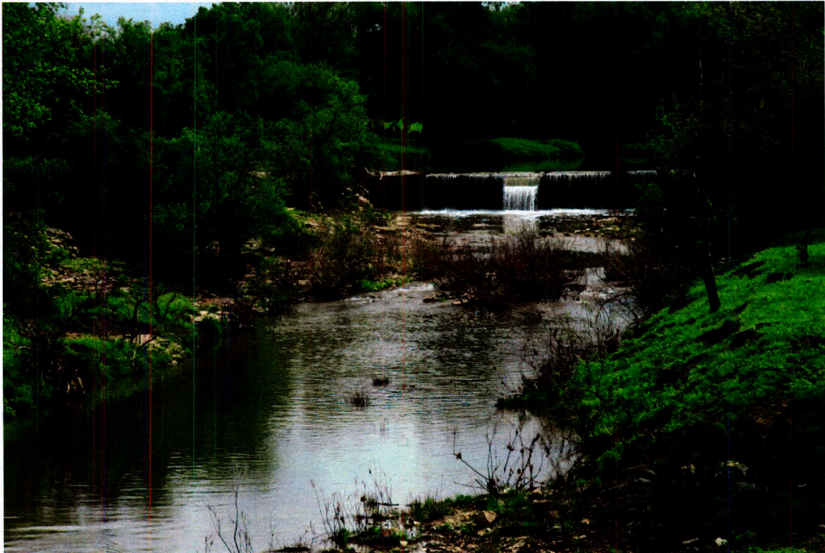
Figure 7.26. Thousands of low head concrete dams have been built on Texas creeks. These dams disrupt the natural movement of sediment that is needed downstream to build point bars and sinuosity. Erosion is often accelerated below the dams, creating additional problems. Some landowners are now considering the removal of these dams. Photo courtesy of Ricky Linex, NRCS.
