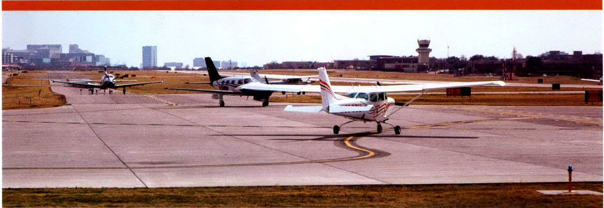
At Addison Airport, two new concrete aircraft holding bays were constructed on both ends of Taxiway Alpha. The north aircraft holding bay capacity was increased by 35 percent compared to the existing holding bay configuration.
