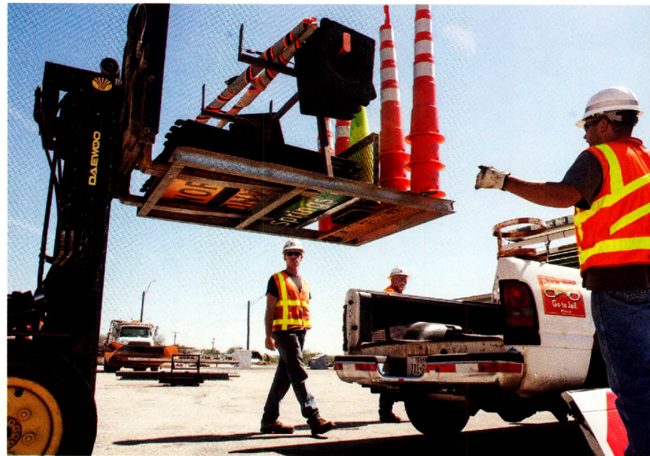
Maintenance Technicians Cody Coltharp (left), Ronney Stone (middle) and Craig Hostas (right) help guide pallets the crew created to speed up and organize truck loading.
