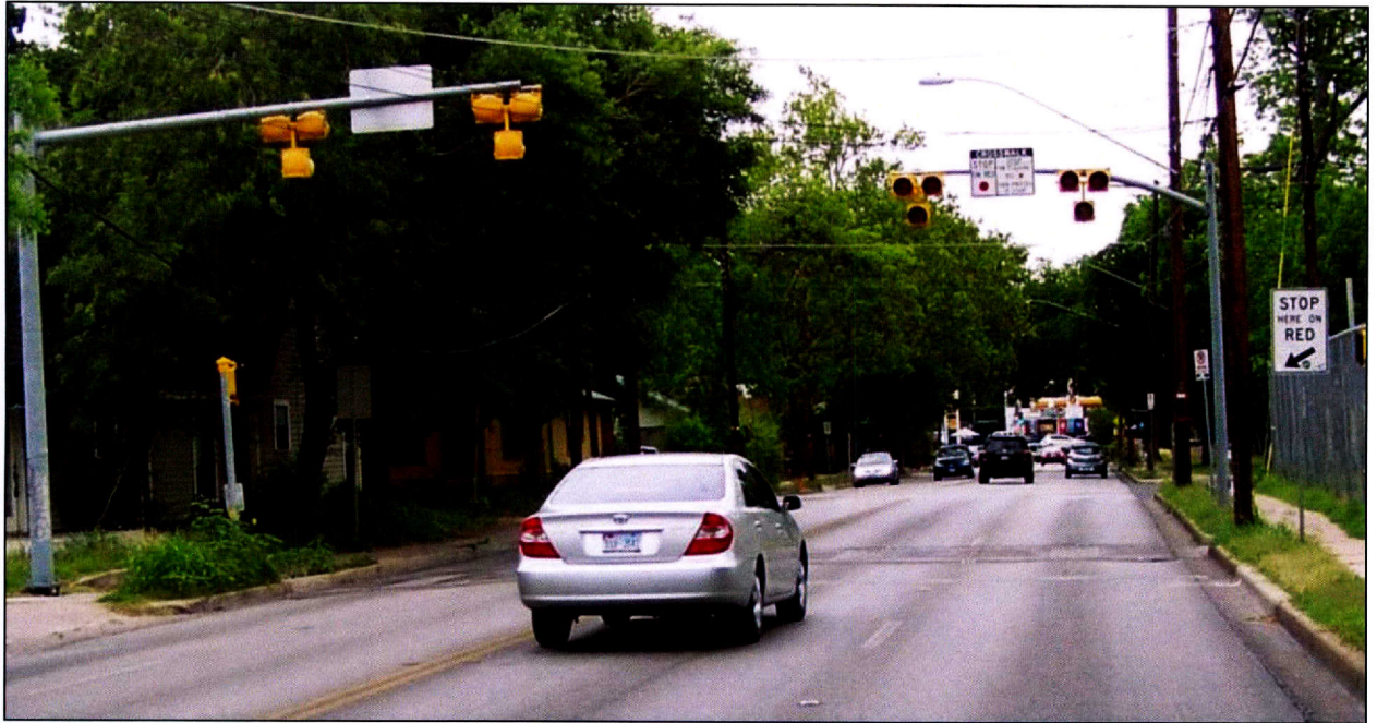
Figure 7. Example of Pedestrian Hybrid Beacon Installation.
