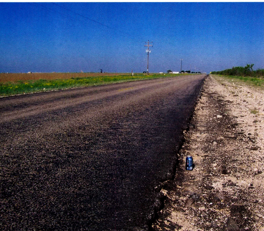
Dangerous failure at the edge of the pavement is caused by traffic loads. One of the technical briefs developed by TxDOT and TTI researchers focuses on shoulder repair techniques.
