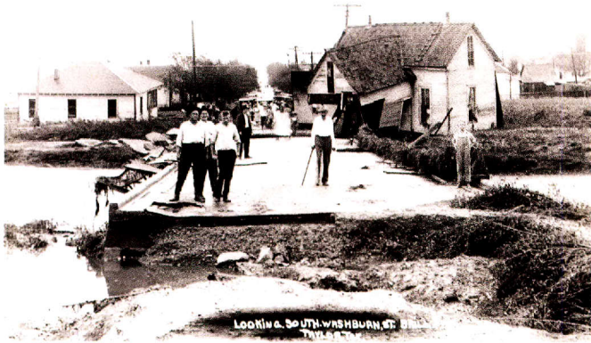
Looking South Washburn St.
