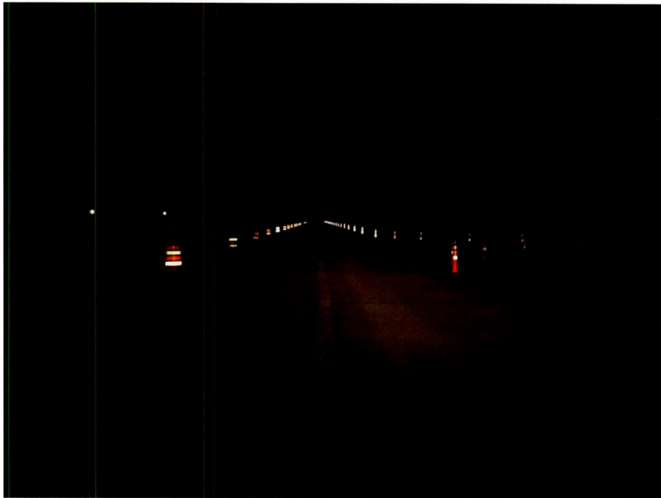
Figure A-32. Treatment 1: 42-Inch Cones on Main Lane with 42-Inch Cones on Driveway.
