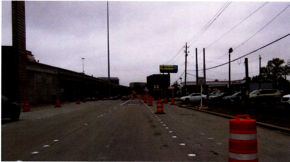
Figure 18. Typical Work Zone Setup at Houston Driveways.
