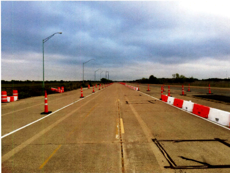
Figure A-28. Treatment 6: 18-Inch LCDs on Main Lane with 42-Inch Cones on Driveway.
