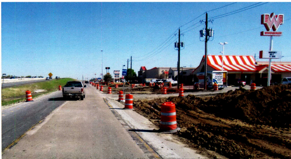
Figure 17. Typical Work Zone Setup at McKinney Driveways.
