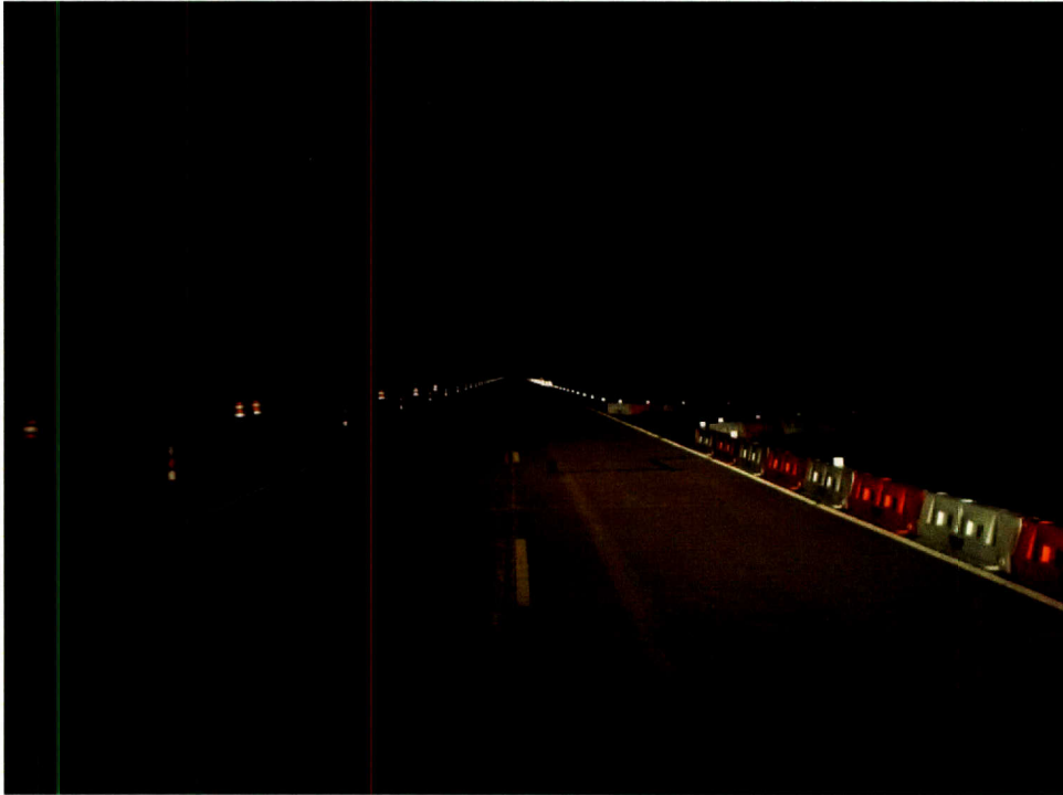
Figure A-39. Treatment 8: 18-Inch LCDs on Main Lane with 18-Inch LCDs on Driveway.
