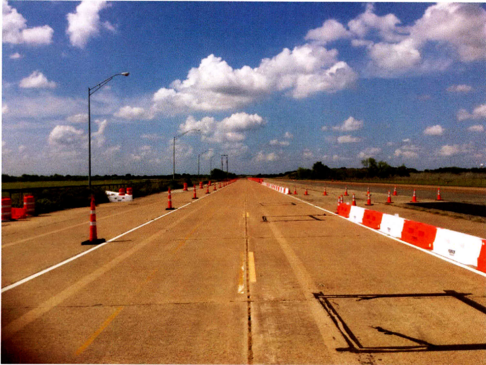
Figure A-29. Treatment 7: 18-Inch LCDs on Main Lane with 28-Inch Cones on Driveway.
