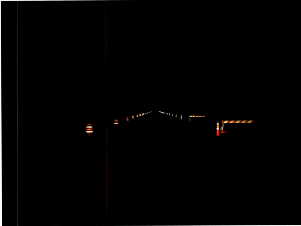
Figure A-35. Treatment 4: 42-Inch Cones on Main Lane with 36-Inch Type I Barricades on Driveway.
