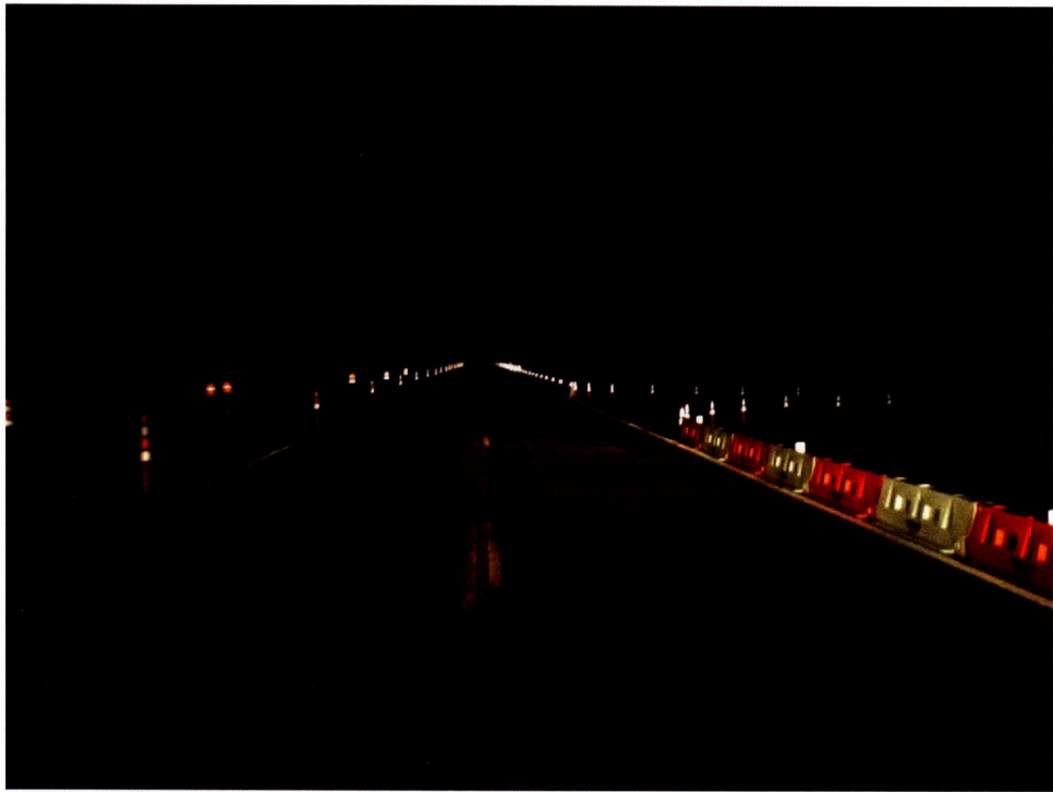
Figure A-38. Treatment 7: 18-Inch LCDs on Main Lane with 28-Inch Cones on Driveway.
