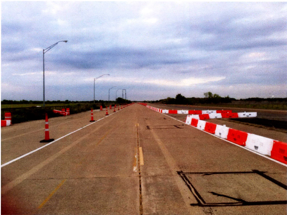
Figure A-30. Treatment 8: 18-Inch LCDs on Main Lane with 18-Inch LCDs on Driveway.
