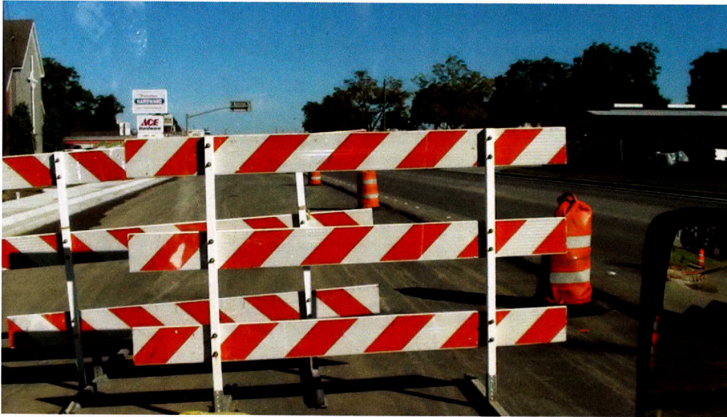
Figure 5. Type 3 Barricades in a Texas Work Zone.
