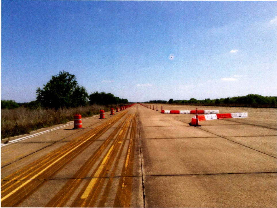
Figure A-25. Treatment 3: 42-Inch Cones on Main Lane with 18-Inch LCDs on Driveway.
