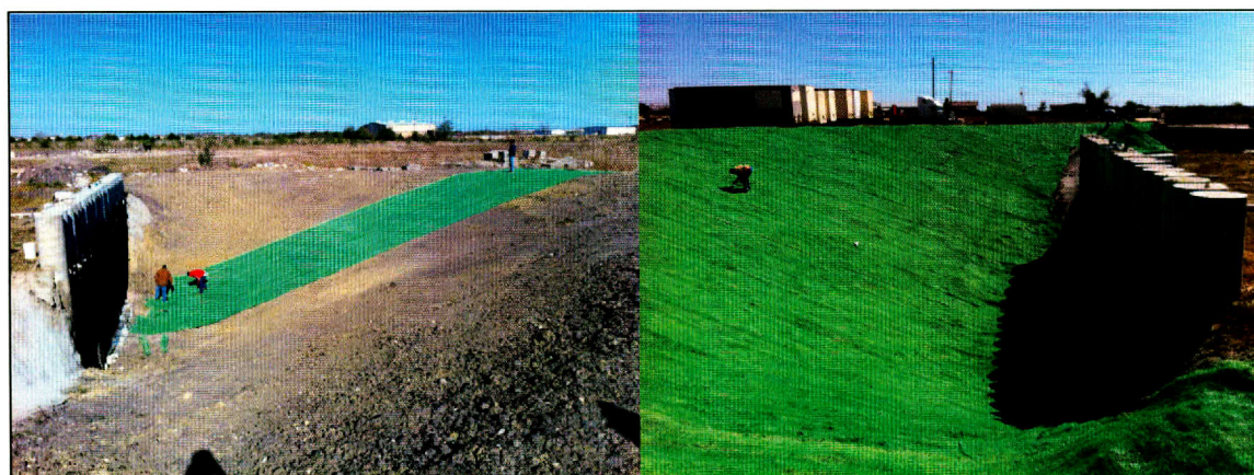
Figure 4.21: Erosion control material is installed on October 18, 2011.
