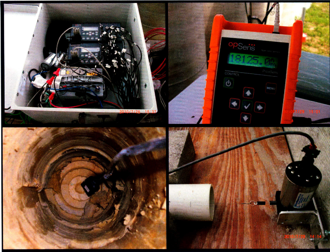
Figure 4.13: Instrumentation on the project site.
