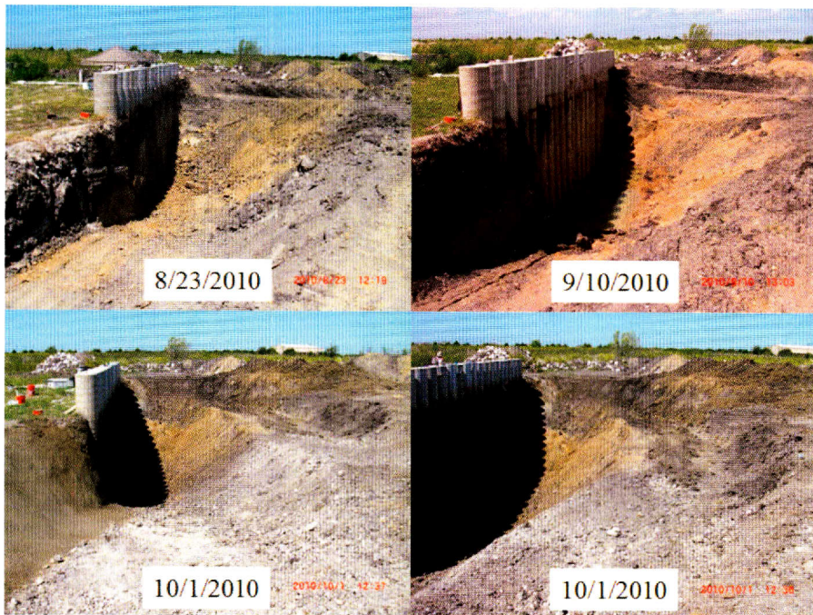
Figure 5.6: Photos of later excavation progress (8/23/2010 - 10/1/2010).
