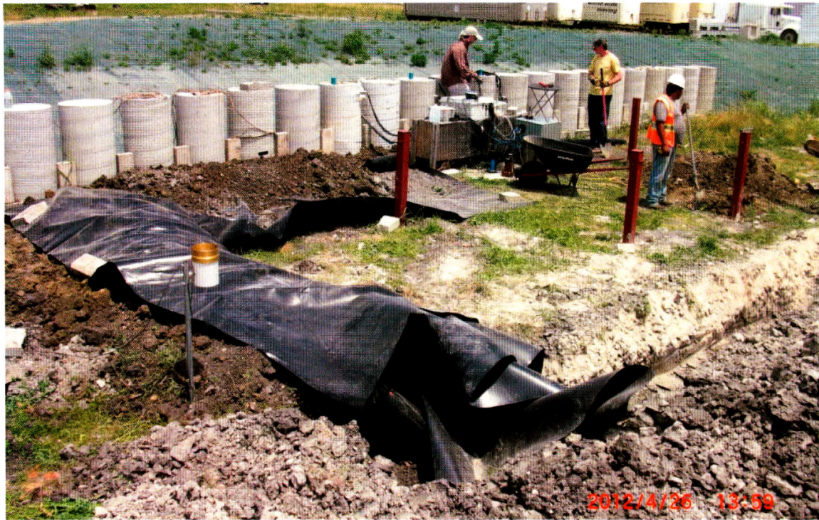
Figure 4.30: Installation of geomembrane in trench.
