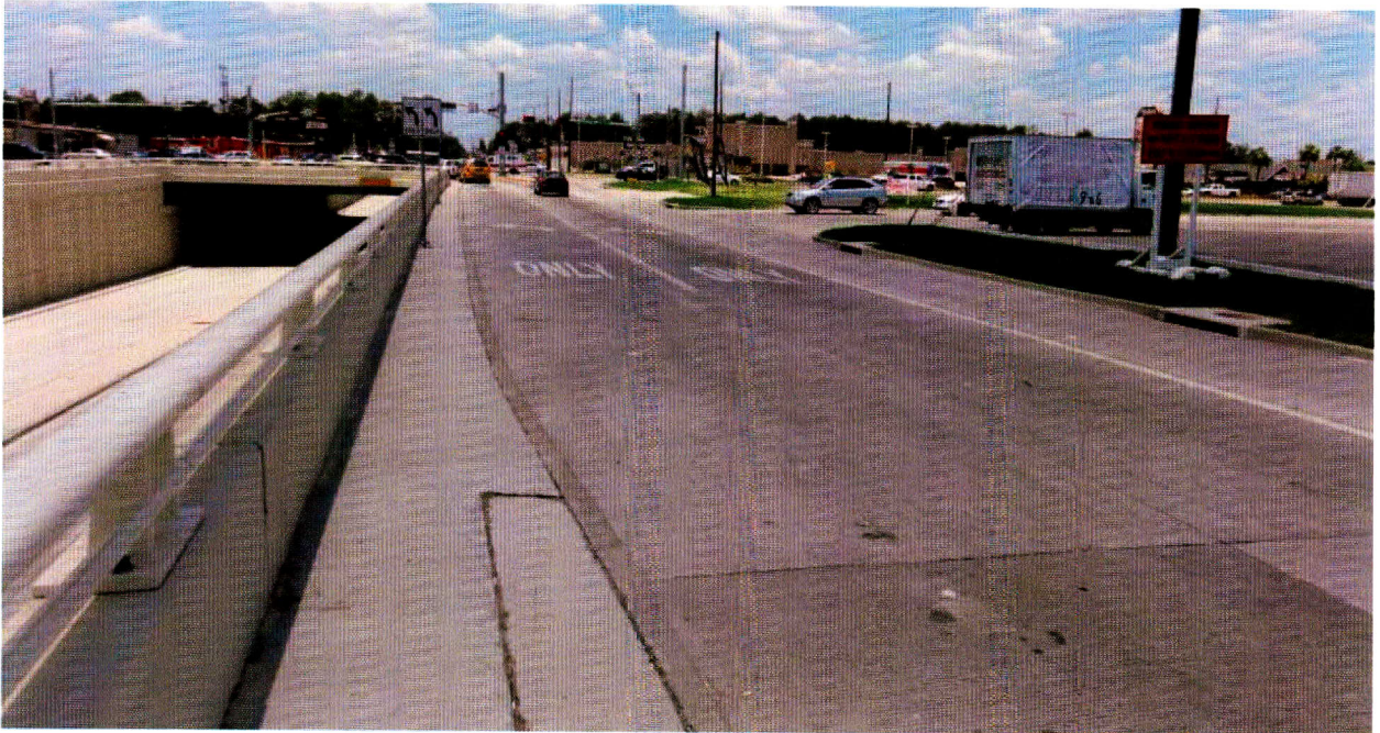
Figure 3.28: Paved area behind the wall. In all locations, pavement extends at least 30 feet behind the wall.
