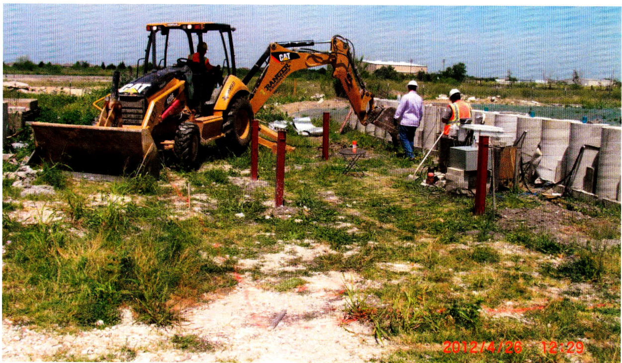
Figure 4.29: Excavation of trench for inundation berm.
