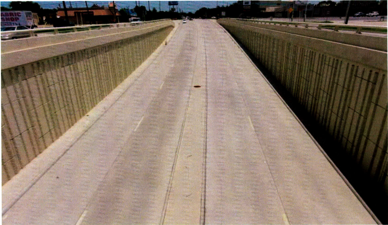
Figure 3.26: View of north and southbound walls from FM 1960 bridge (facing southeast).
