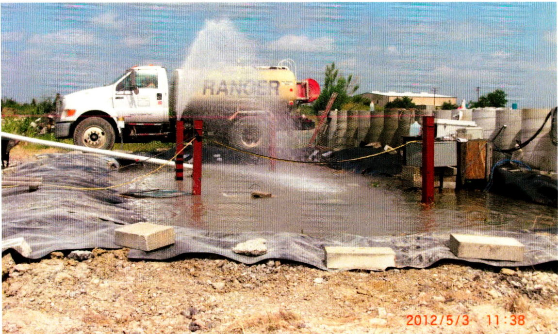
Figure 4.35: Filling the inundation zone.
