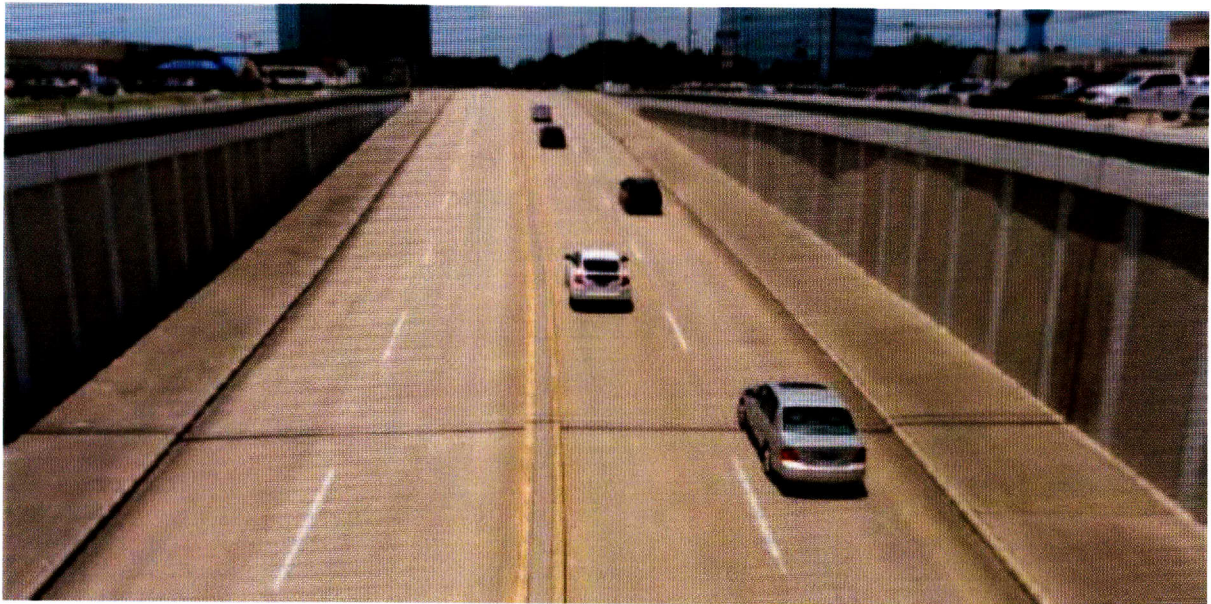
Figure 3.35: View of current wall conditions, facing west.
