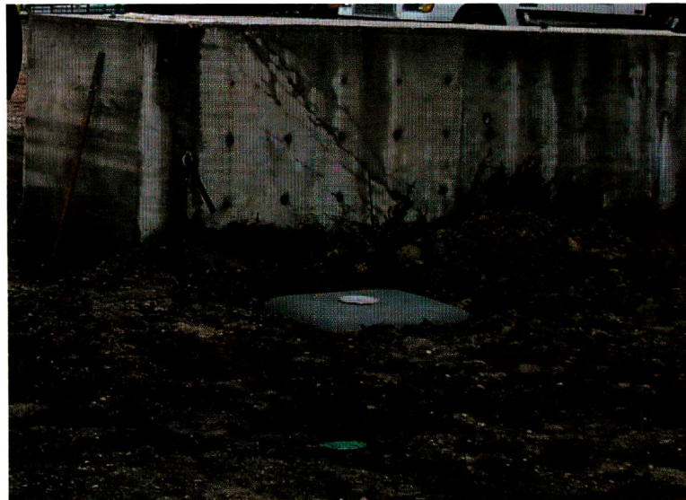
Figure 4.24: The piezometer installed and covered in borehole B-3.
