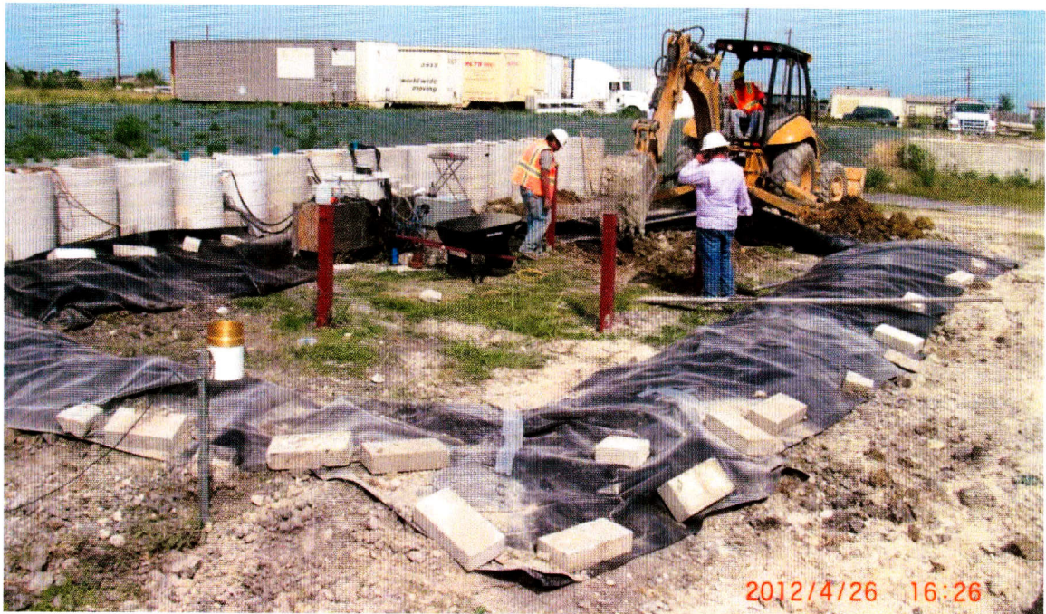
Figure 4.32: Compacting soil with backhoe bucket.
