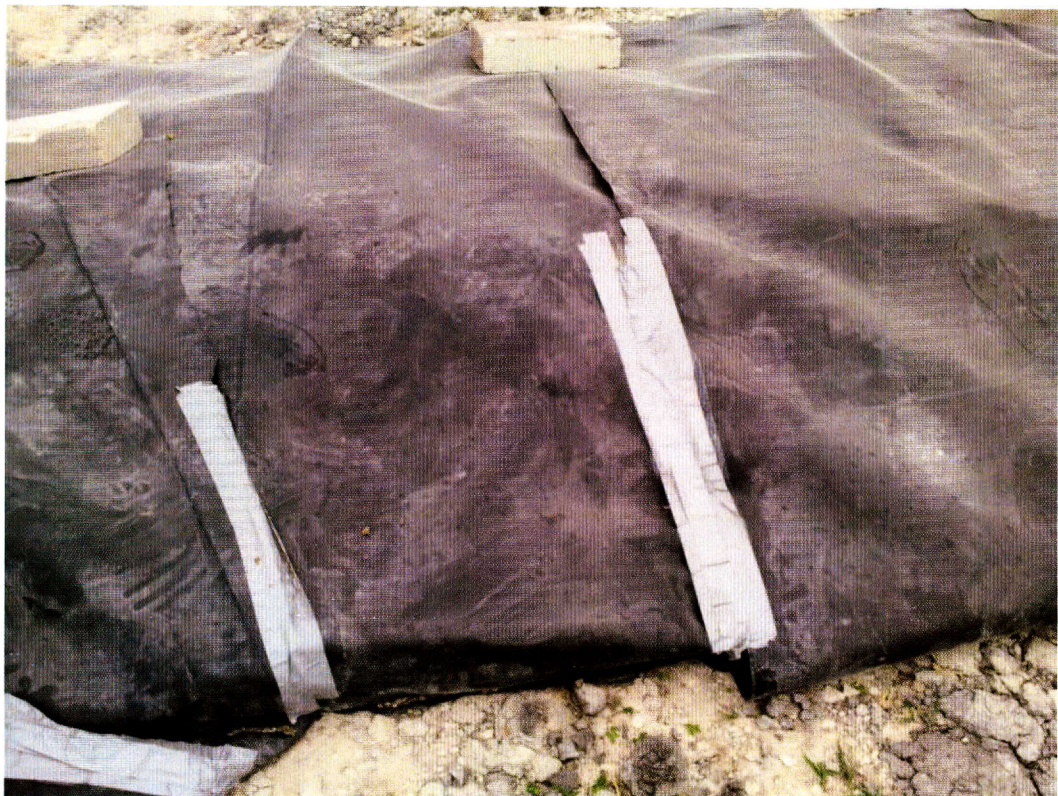
Figure 4.33: Detail of geomembrane seam.
