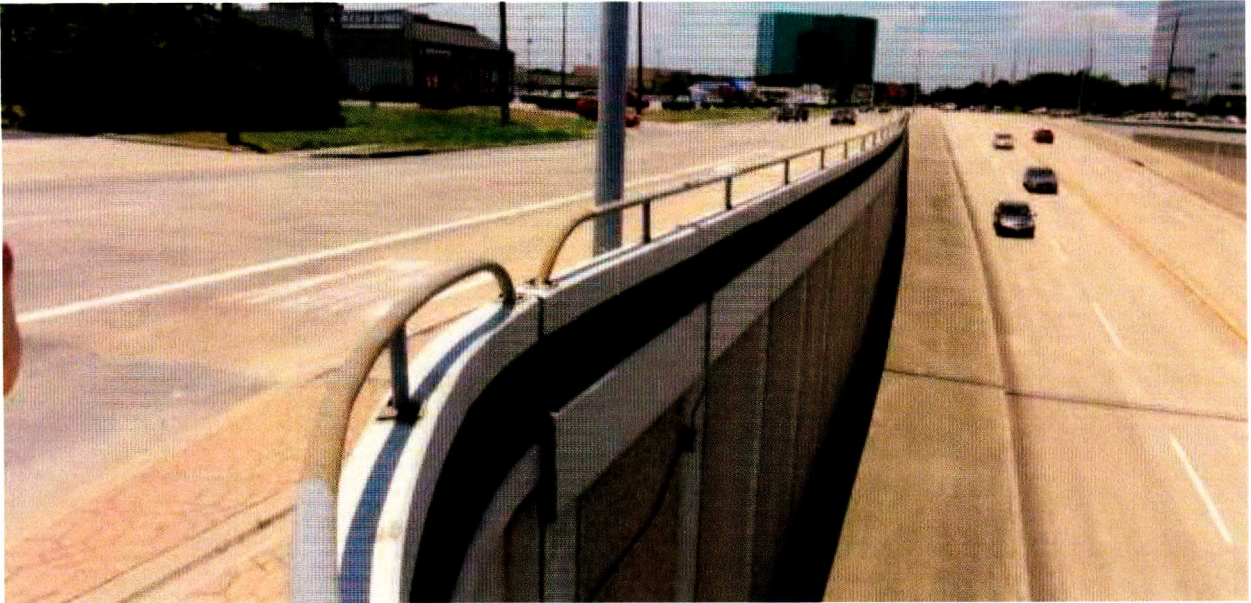
Figure 3.39: View of pavement coverage along southwestern side of intersection (facing west).
