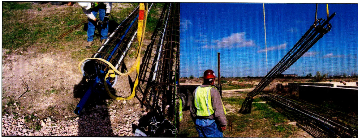
Figure 4.15: Lifting an instrumented cage with two cranes.
