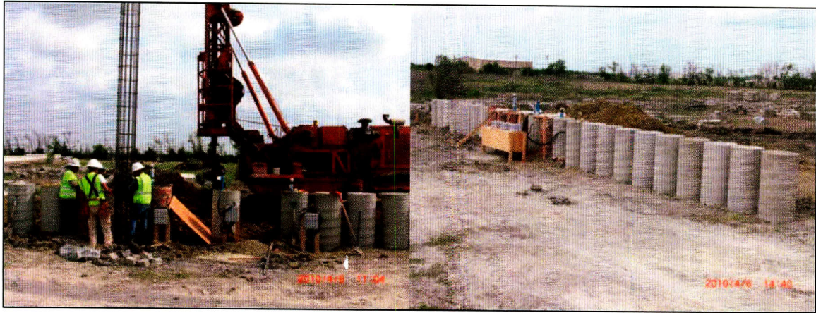
Figure 4.14: Construction of test wall, April 2010.
