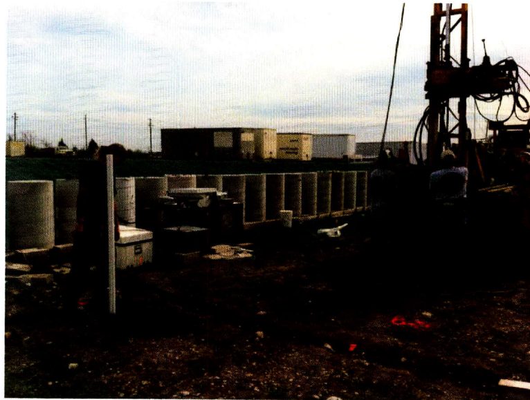
Figure 4.25: Piezometer being installed in borehole A.
