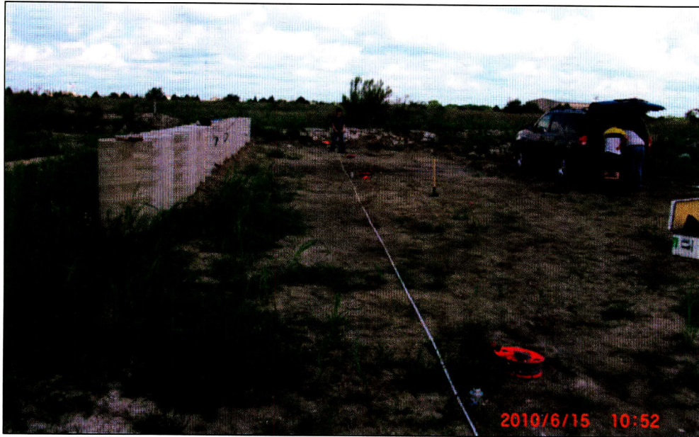
Figure 6.5: SASW testing at the test wall prior to excavation, June 2010.
