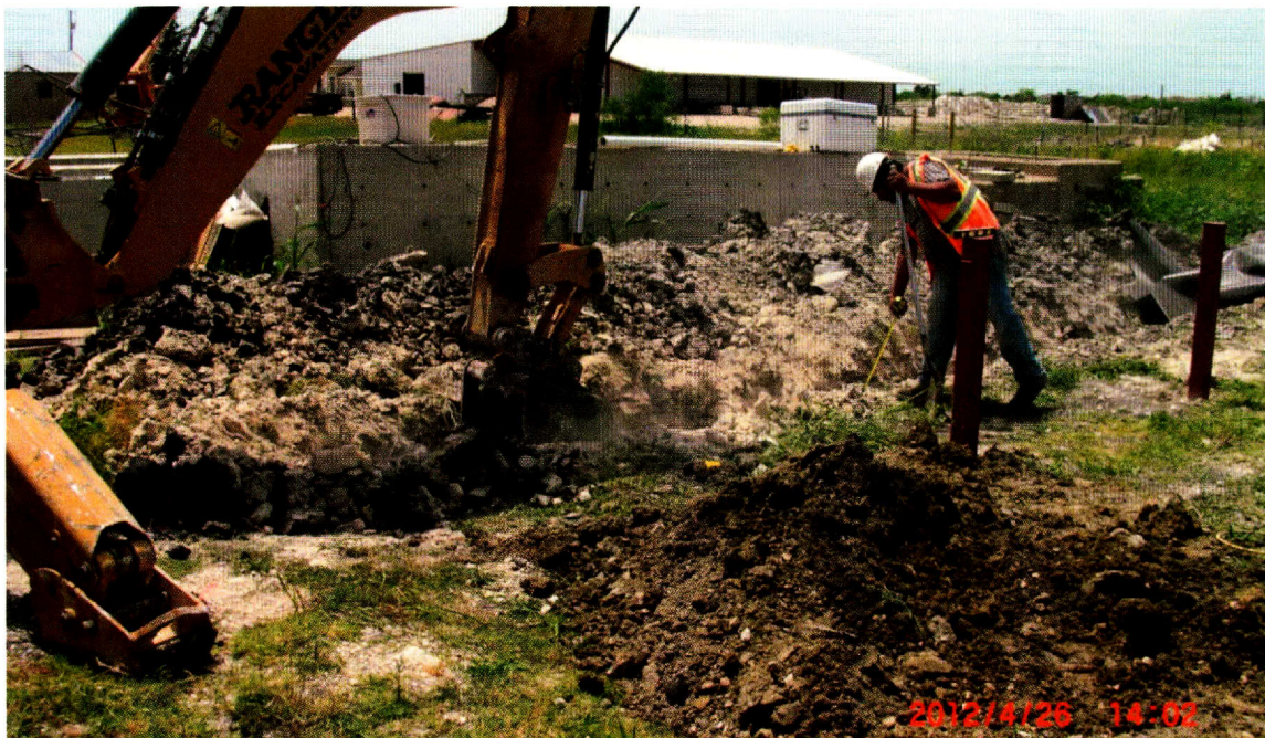
Figure 4.31: Compacting soil with backhoe bucket.
