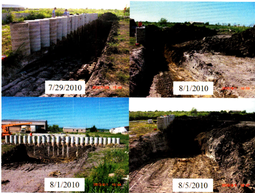
Figure 5.5: Photos of initial excavation progress (7/29/2010–8/5/2010).
