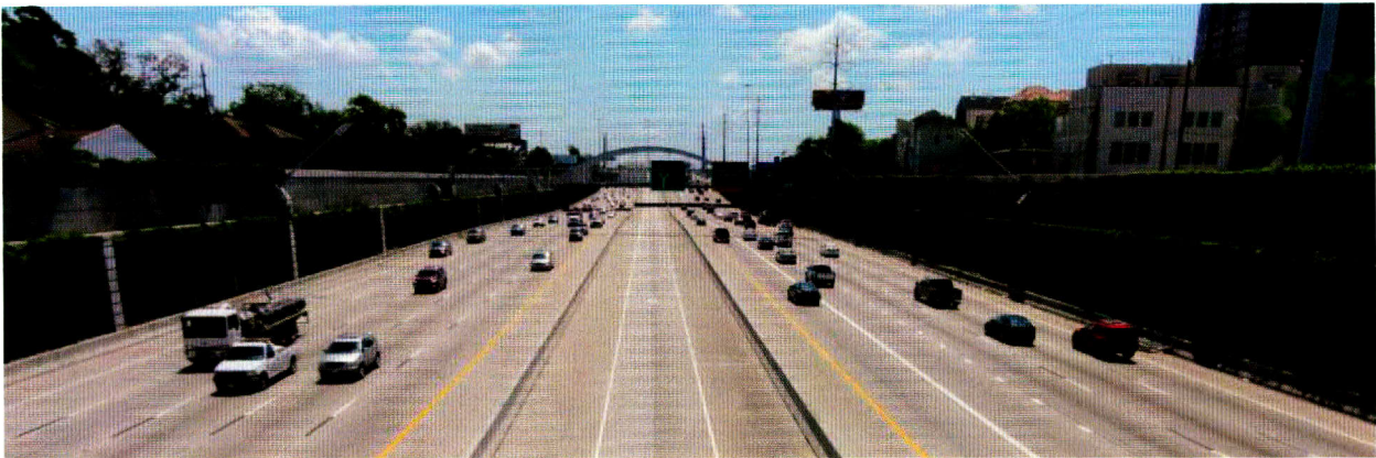
Figure 3.31: Large-scale view of project area (facing east). Sound wall is located above the main retaining structure.
