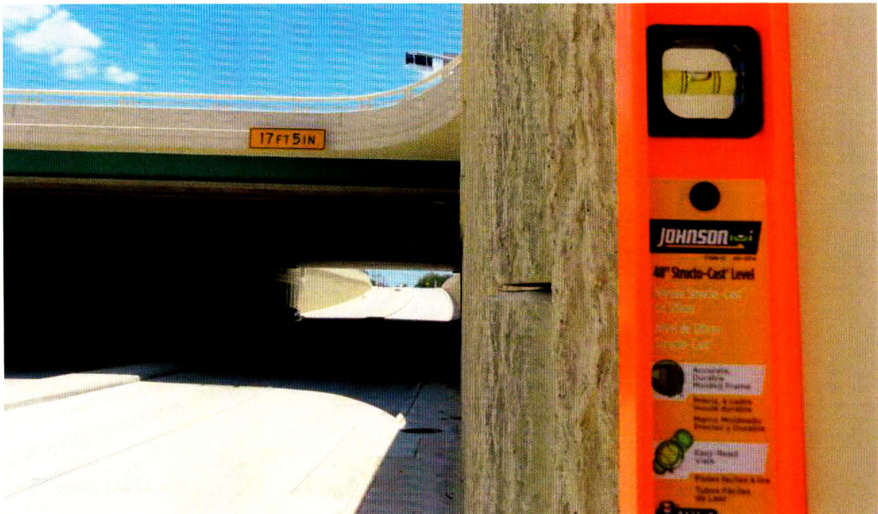
Figure 3.27: Wall facing was observed to be vertical and in good condition throughout the project area.
