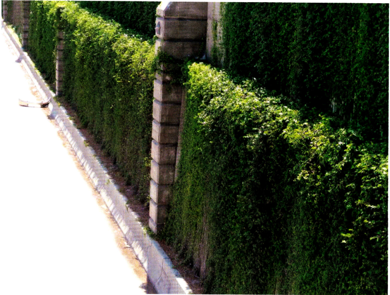
Figure 3.32: Dense vegetation and batter angle on concrete facing panels. Sound wall is located above main retaining structure.
