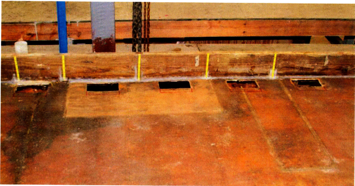
Figure B-12 6in. × 8in. Drain Placement
