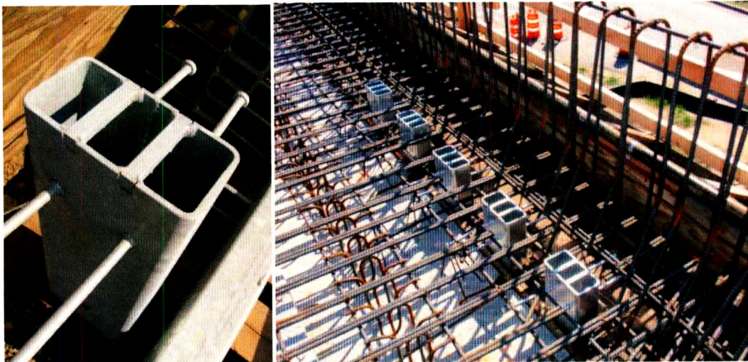
Figure 1-1 New Type of Rectangular Deck Drain (Pictures Provided by TxDOT)
