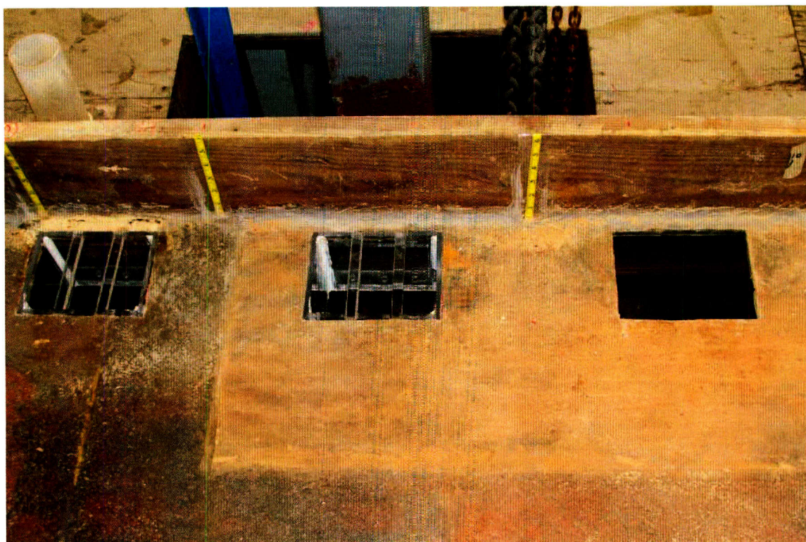
Figure B-14 6in. × 8in. Drain Installation
