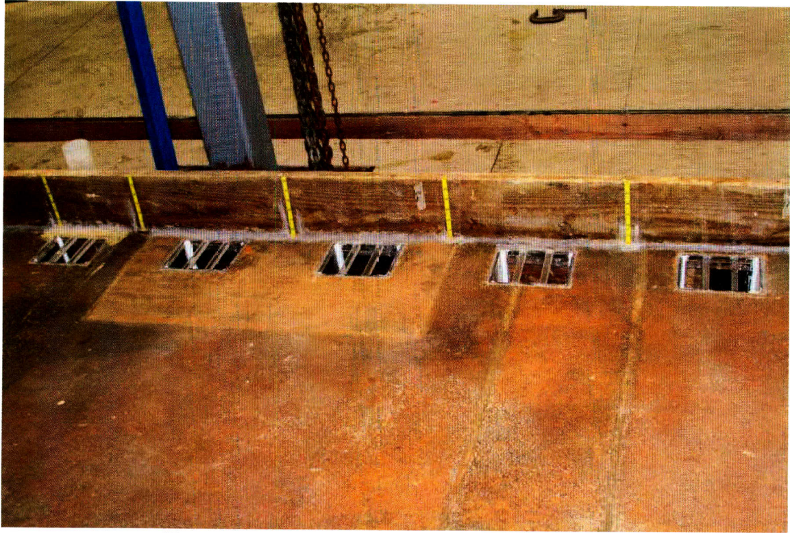
Figure B-15 Finished 6in. × 8in. Drain Installation
