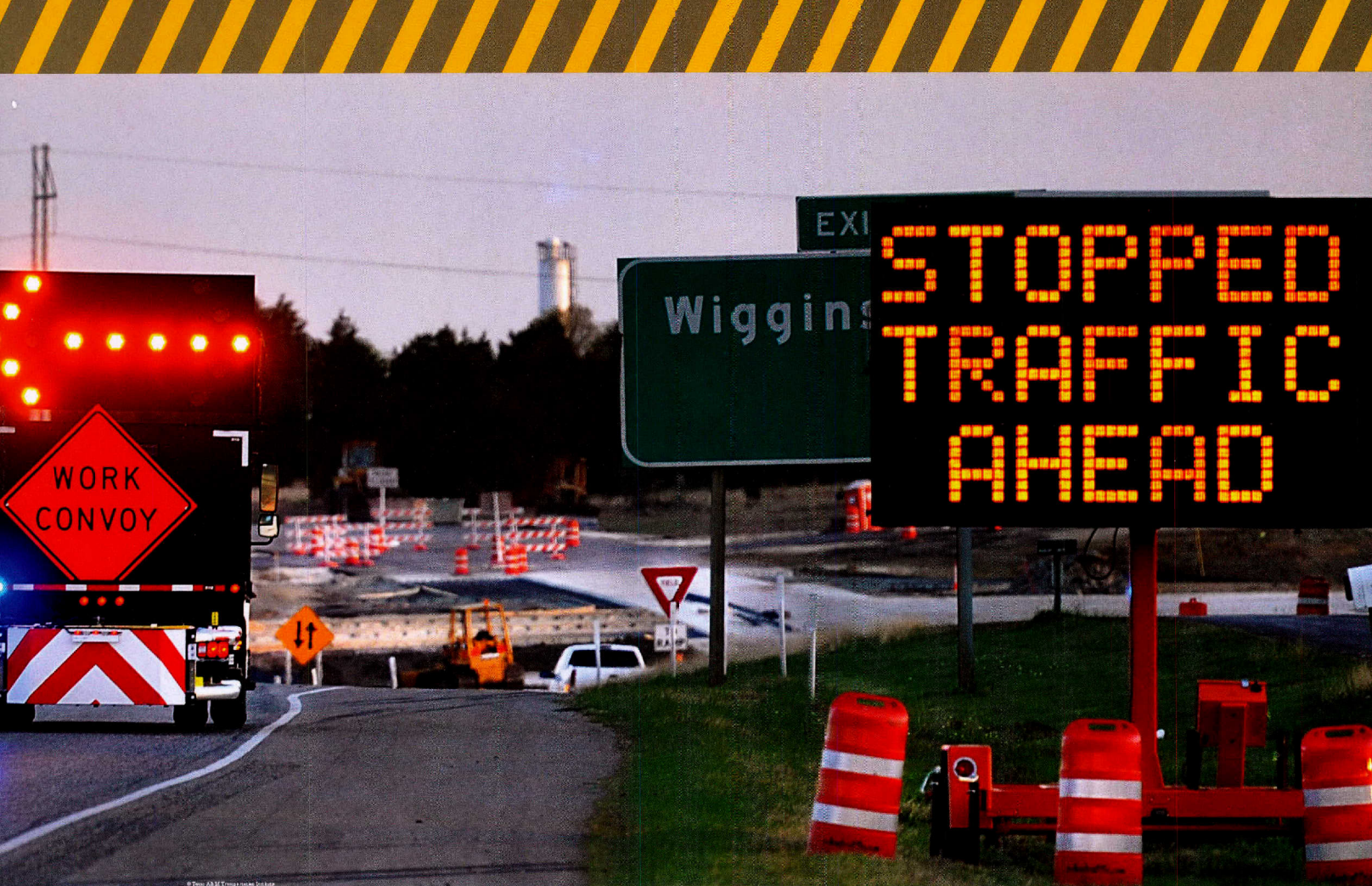
When traffic slows down or stops due to work zone activities on I-35, the end-of-queue warning system developed by TTI for TxDOT informs motorists ahead of time. That means a better chance for drivers to avoid rear-end collisions.
