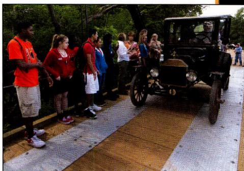
Above and at right: The Piano Bridge in Fayette County was recently preserved thanks to support from county officials and preservationists.
