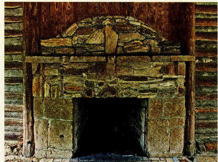
Fireplace, Mission Tejas: Pieces of petrified wood are set in a stylized pattern in this bit of CCC handiwork, one of the decorative touches found throughout CCC parks.
