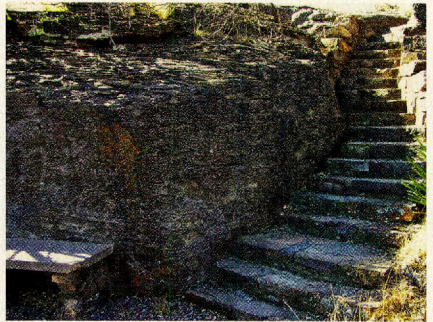
Rock stairway, Davis Mountains: Unless climbers watch their feet as they walk the trail to this Skyline Drive picnic area, they may miss the craftsmanship of this winding stairway the CCC built into the side of the mountain.
