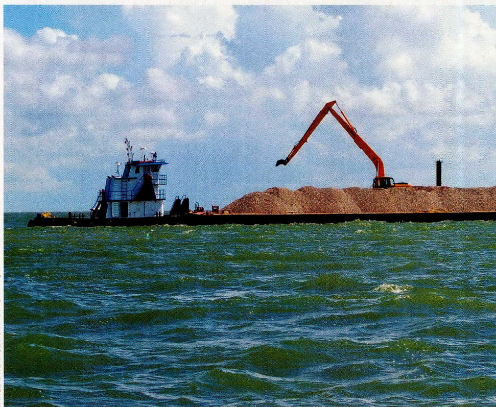
BARGE BY LANCE ROBINSON/TPWD; OYSTERS BY TPWD
