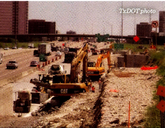
Millions of cubic yards of soil excavated during construction of the LBJ Expressway were recycled for use within the project and in projects in nearby cities.
