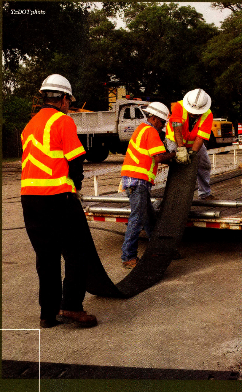
Maintenance crew members in the Austin District load a 105-pound portable rumble strip onto their trailer using the new rumble strip roller invented by staff after a maintenance employee was injured trying to lift the strip onto his trailer.
