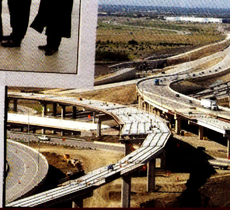
Looking west, DFW Connector construction makes major progress.
