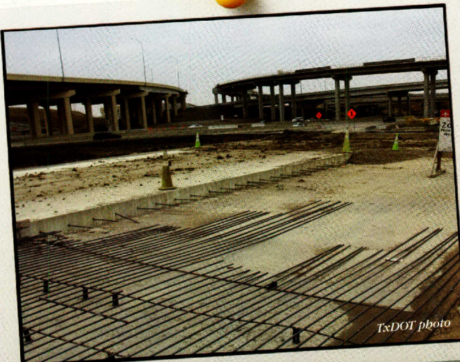
Tons of rebar goes into reinforcing the 1.6 million square yards of concrete needed for this project.
