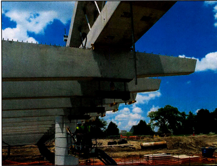
Figure 2.19- Post tensioning the floor beam bars.
