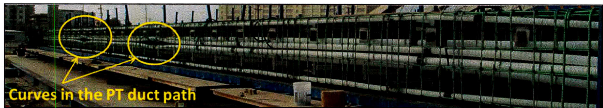
Figure 2.12- Intentional curves in the duct paths.
