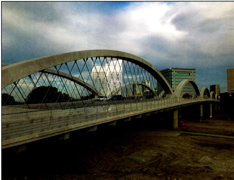
Figure 1.2- The new West 7 th Street Bridge.
