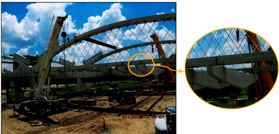
Figure 2.18- Initial hanging of the floor beams.
