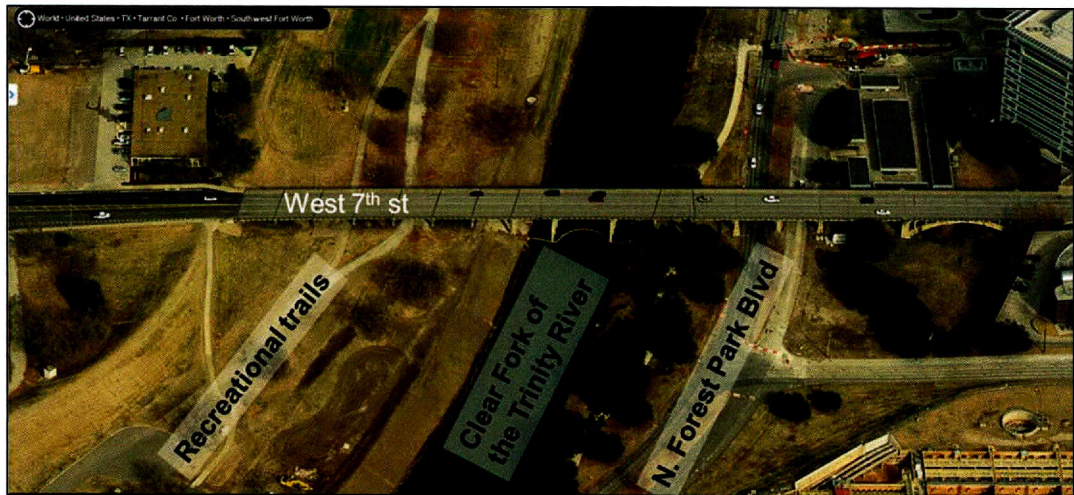
Figure 1.1- The location of the West 7 th Street Bridge [1].
