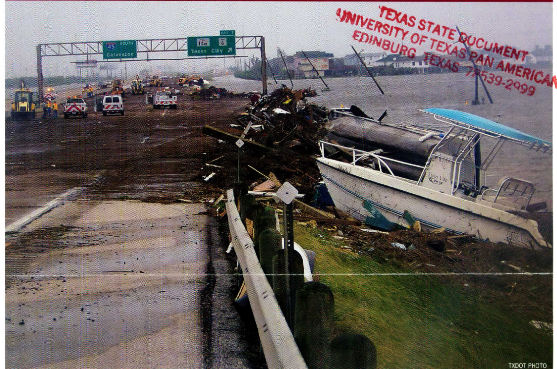
In the aftermath of Hurricane Ike, Texas Department of Transportation's Yoakum and Houston District forces arrive on Interstate 45 for combined cleanup of main lanes leading into Galveston.
