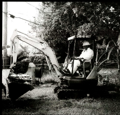
Soil excavation gets under way at 27 residential properties in Corpus Christi after the TCEQ confirmed lead contamination from a nearby industrial facility. The landscaping will be fully restored when cleanup is completed.
