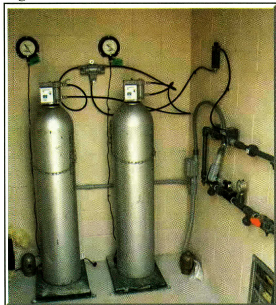
Figure 4b. A Gas Chlorinator
