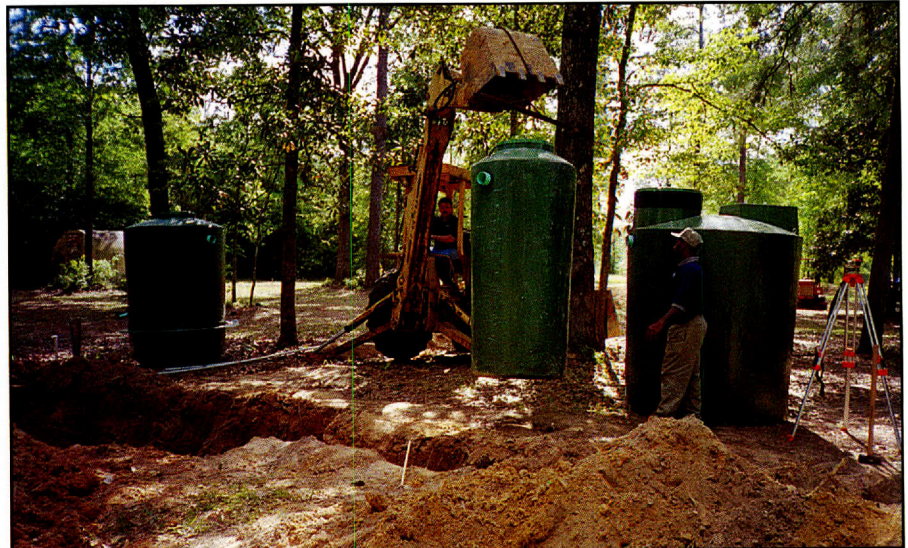
A PRETREATMENT TANK is lowered during installation of an aerobic septic system. The main treatment tank is at right.
