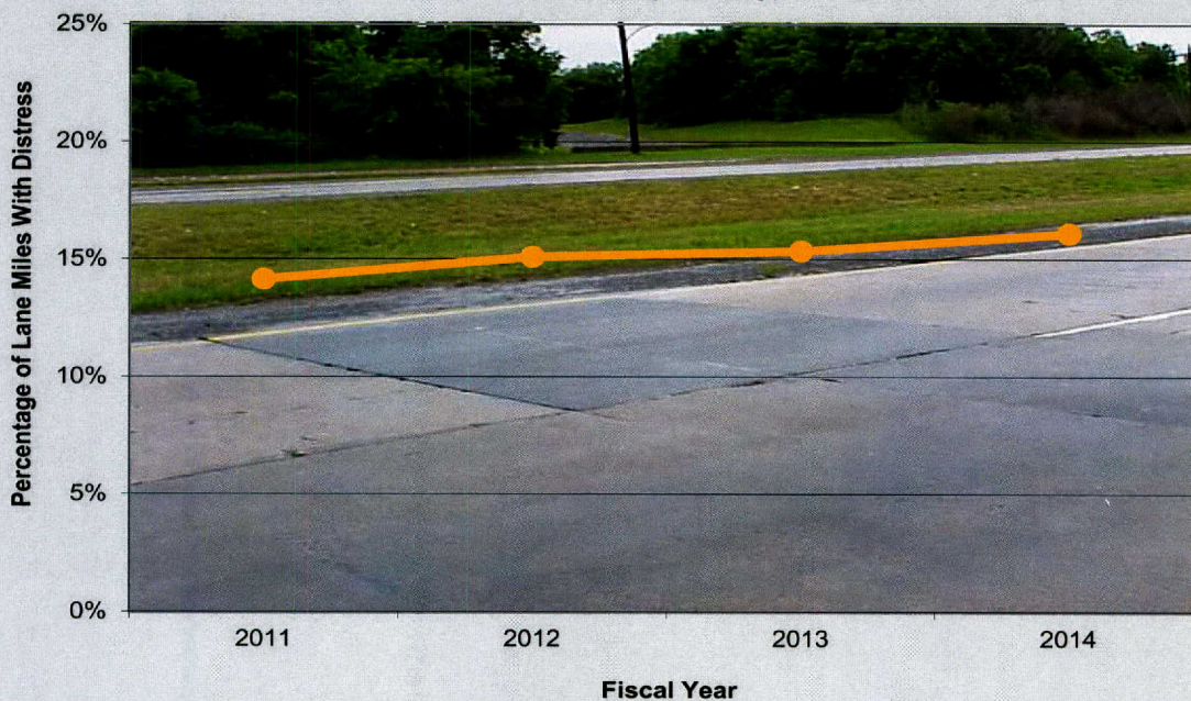
CRCP Concrete Patches (rated), FY 2011–2014
