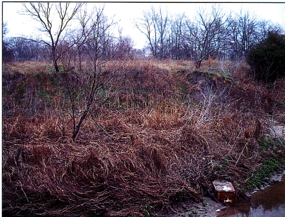
Figure 4. Southernmost stabilization location. View is to the southeast.
