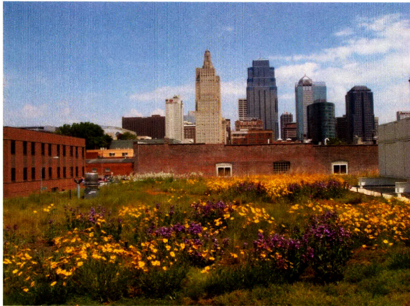
Figure 8: Green Roof at Kansas City, Missouri Public Library Source: Watearth, Inc.
