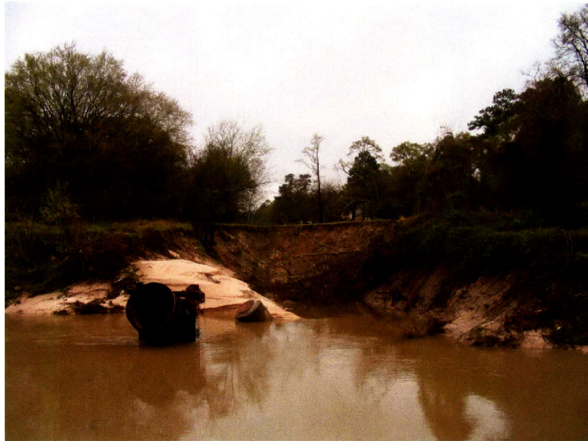
Figure B2: Cypress Creek at Meyer Park – Phase 1, South Bank, Pre-Construction
