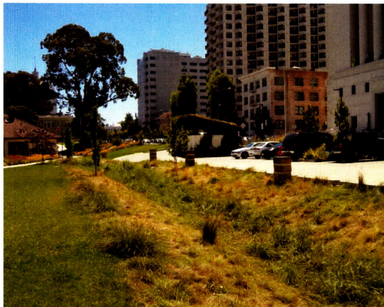
Figure 9: Vegetated Swale at Lake Merritt, Oakland, California Source: Watearth, Inc.
