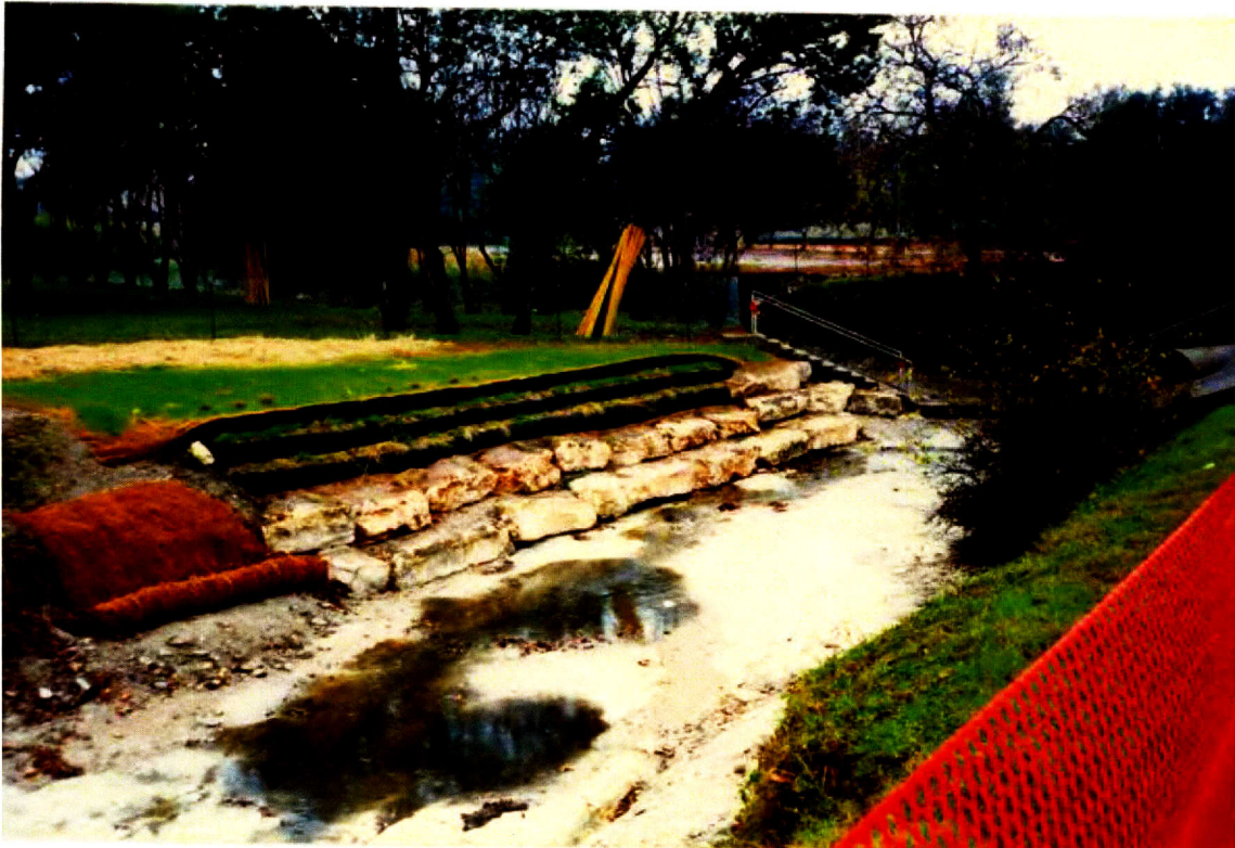
Figure 15: City of Austin Typical Stacked Boulder Wall Installation
