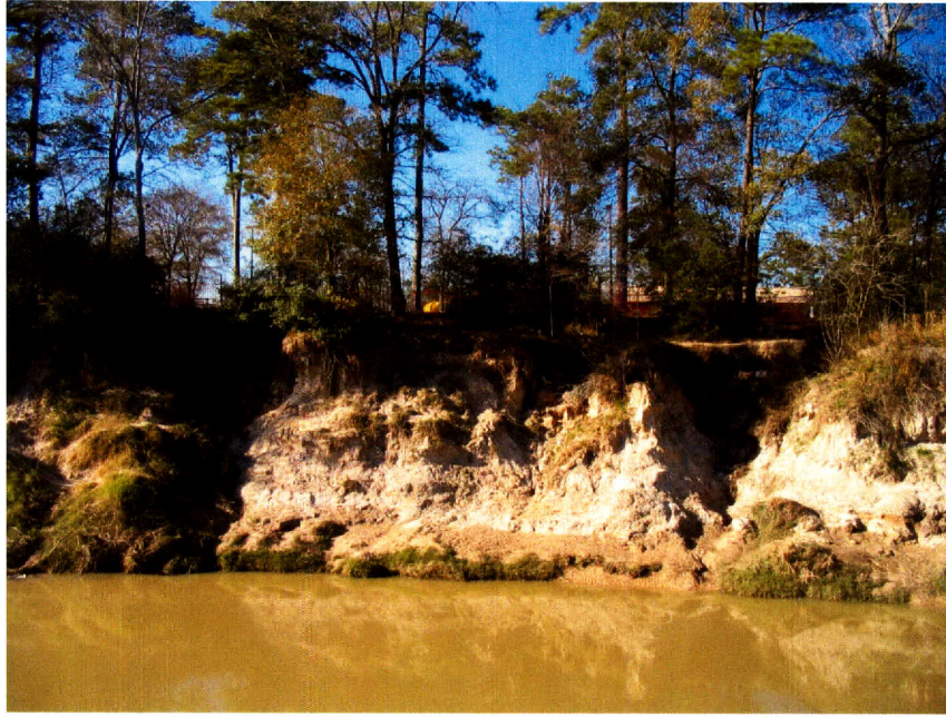
Figure B1: Cypress Creek at Meyer Park – Phase 1, North Bank, Pre-Construction
