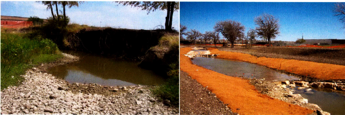
Figure 13: Typical Erosion at East Salitrillo Creek Prior to Construction (left) and View of Project During Construction (right).
