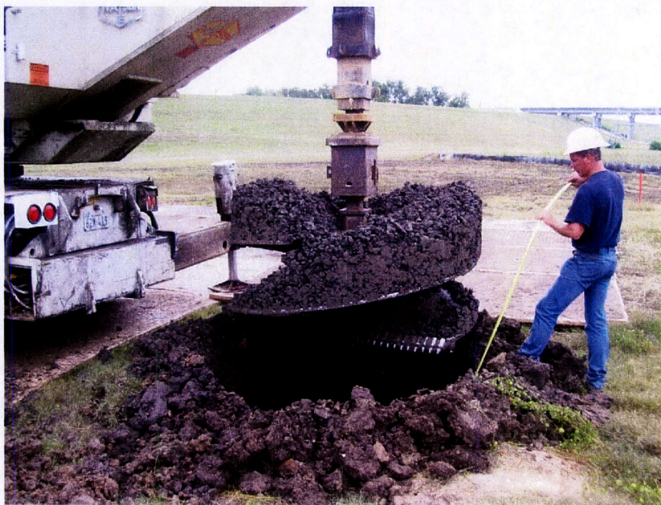
Figure 12. Structure 7/4 showing removal of third alluvial unit, facing south.
