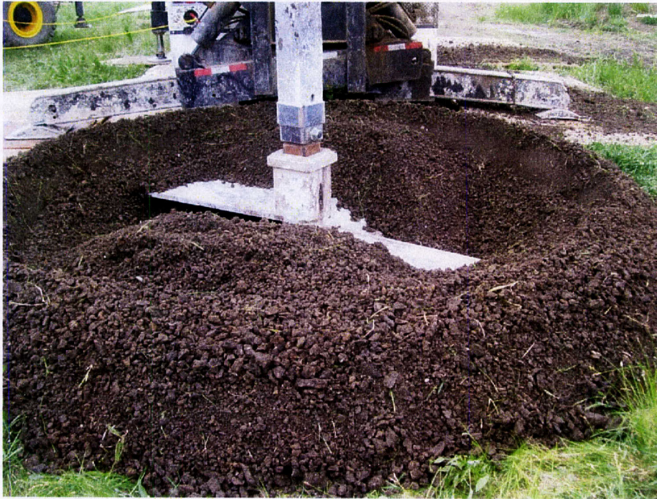
Figure 10. Structure 7/5A showing augering of recent alluvial clay underway, facing southeast.
