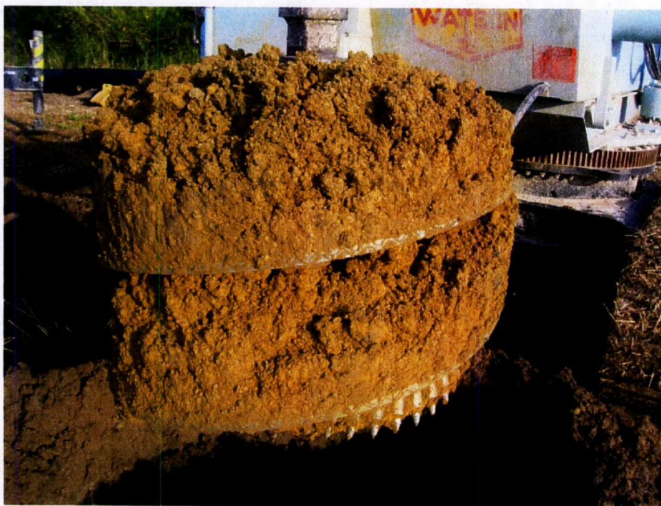
Figure 9. Structure 2/3 foundation hole showing removal of earlier alluvial unit, facing northwest.
