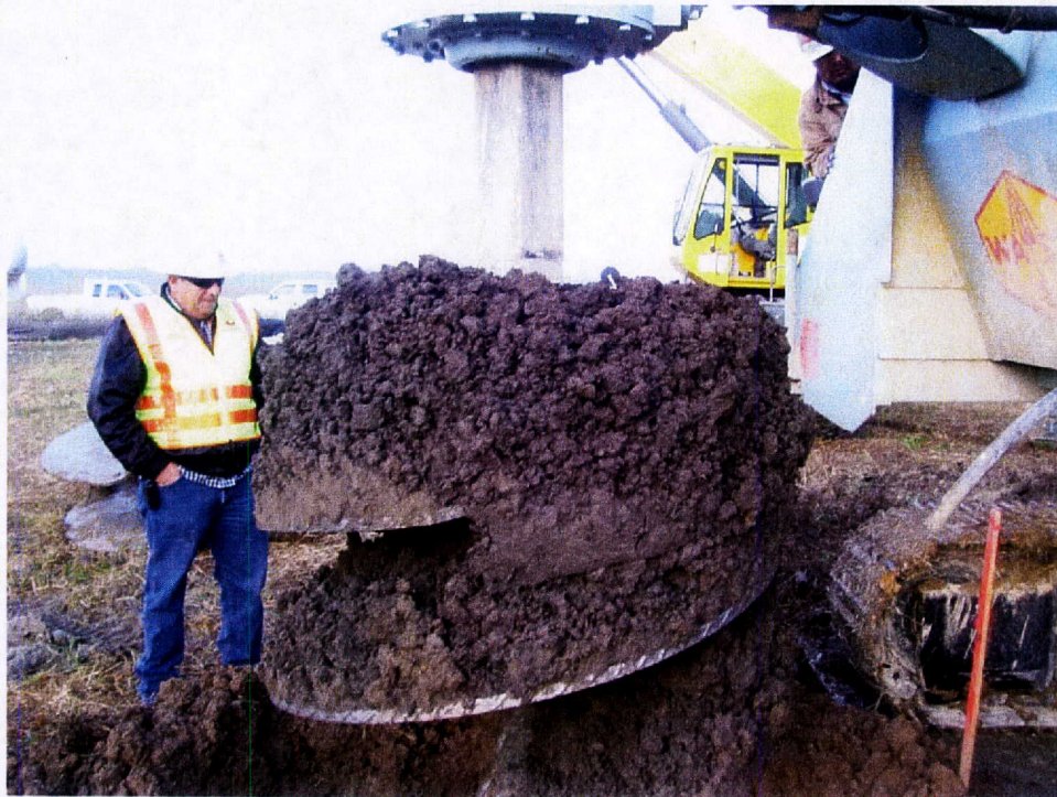
Figure 8. Structure 2/3 foundation hole showing removal of Pilot Point alluvium, facing west.
