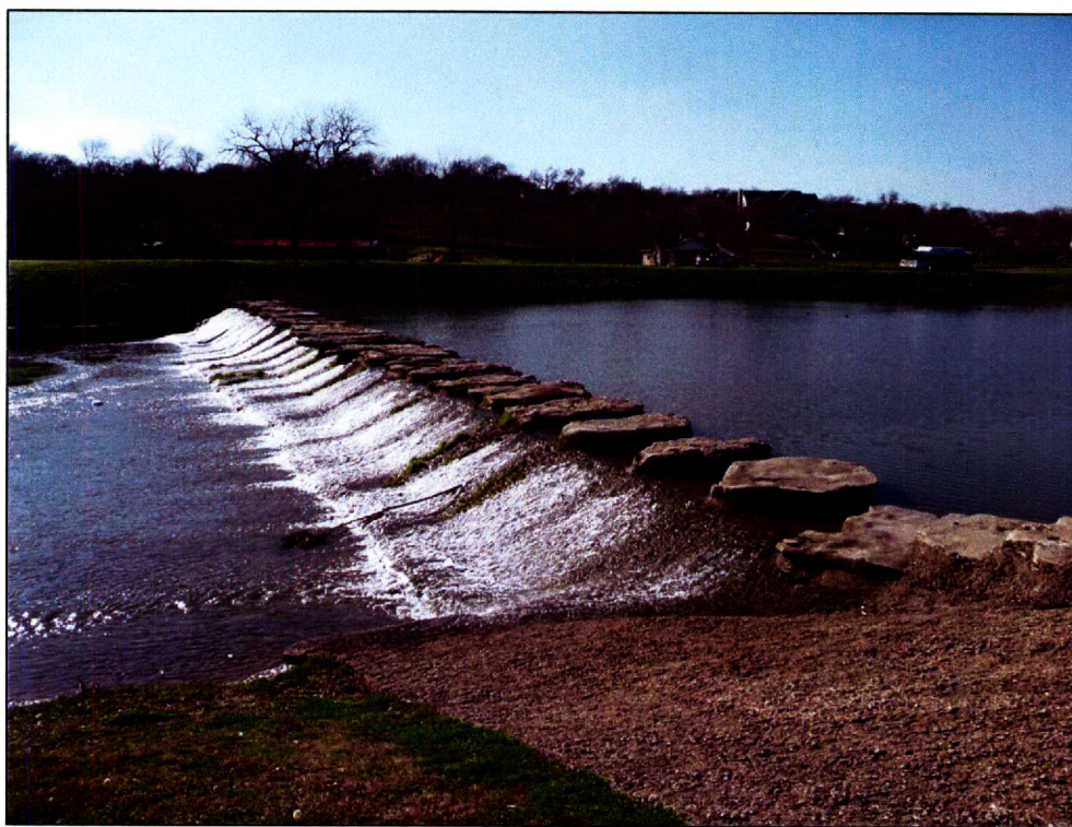
Figure 12. Check dam in Marine Creek Linear Park North, facing west.
