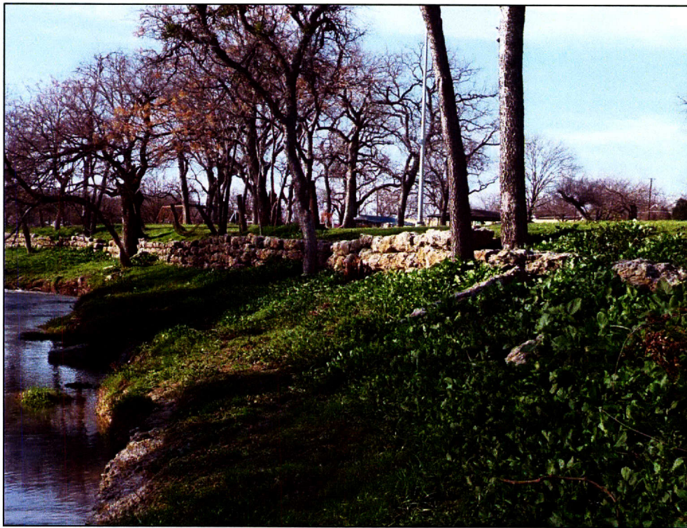
Figure 14. Overview of large rock pilings along Marine Creek in Lincoln Park, facing north.
