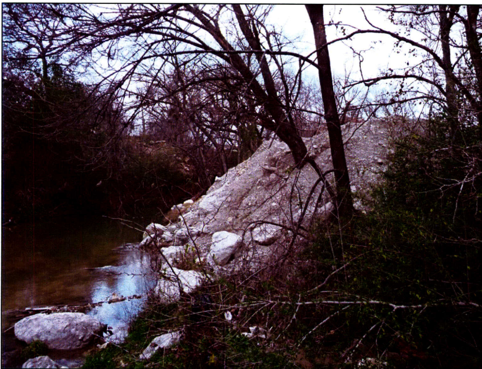
Figure 4. Spoils pile eroding into Marine Creek north of Buck Sansom Park. Beyond north/northwestern boundary of Buck Sansom Park, facing north/northwest.
