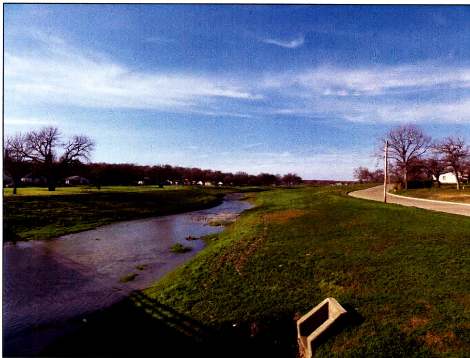
Figure 6. Overview of typical modified topography along park corridor, notice buried culvert in foreground and leveled areas for roadways along both side of Marine Creek. Photo is facing north from NW 30 th Street.
