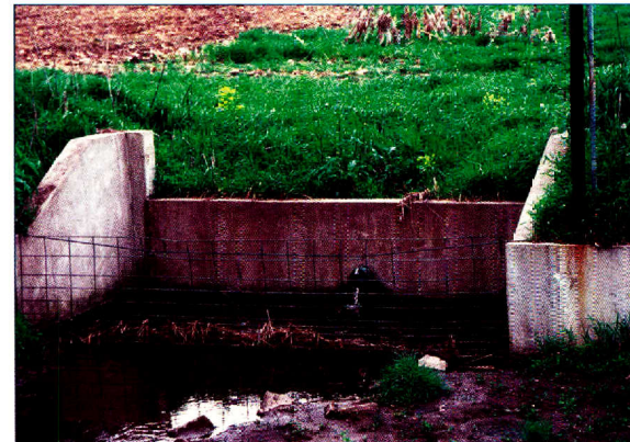
Figure 6. Grade stabilization structure. (Source: USDA–NRCS)
