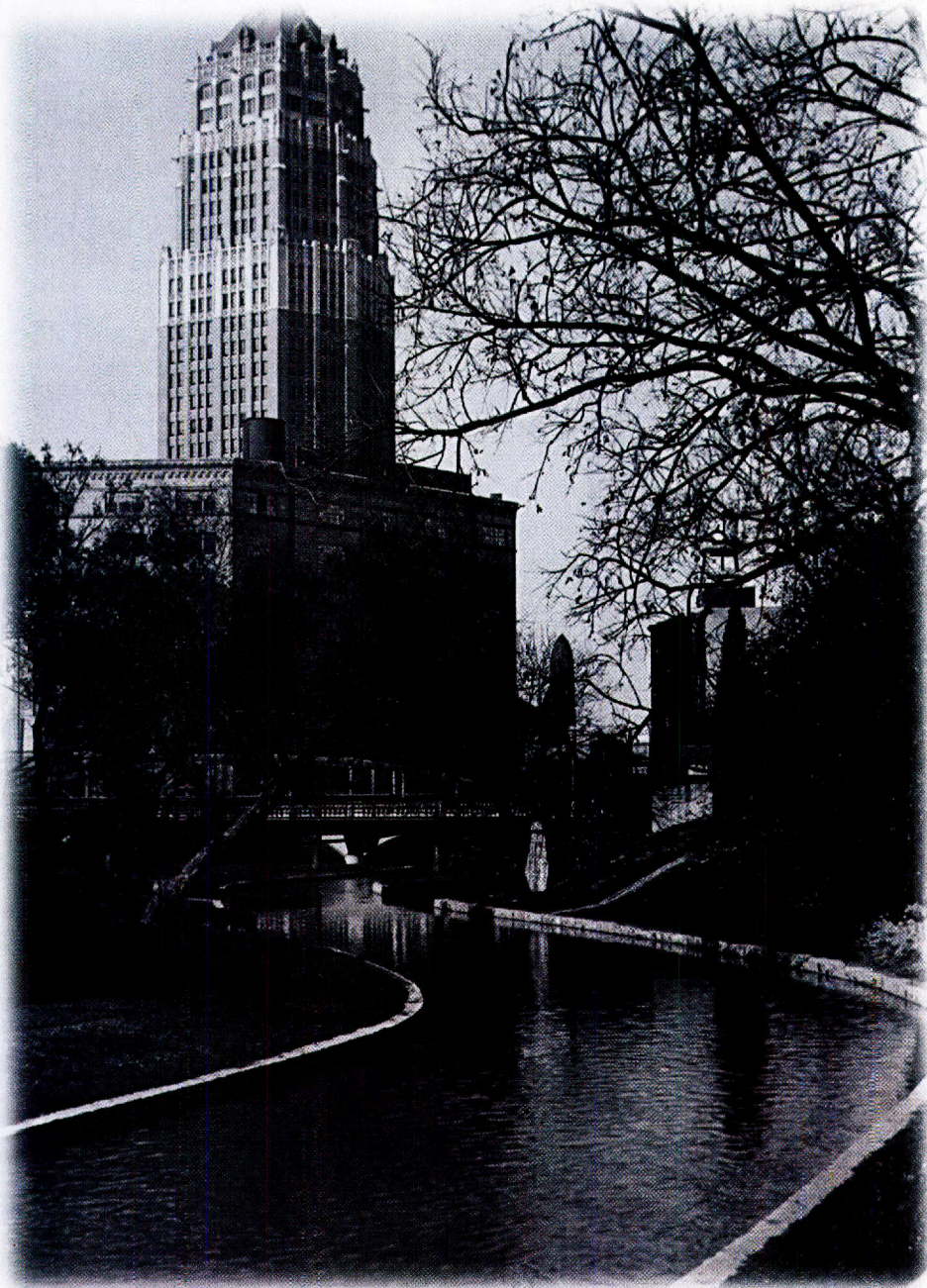
In 1929, Robert Hugman presented the city with a redesign of Surkey's River Walk. Hugman's project, which straightened this bend (shown here in 1930), finally began in 1939, finished in 1941, and earned him the title "Father of the River Walk." PHOTO COURTESY LEWIS F. FISHER
