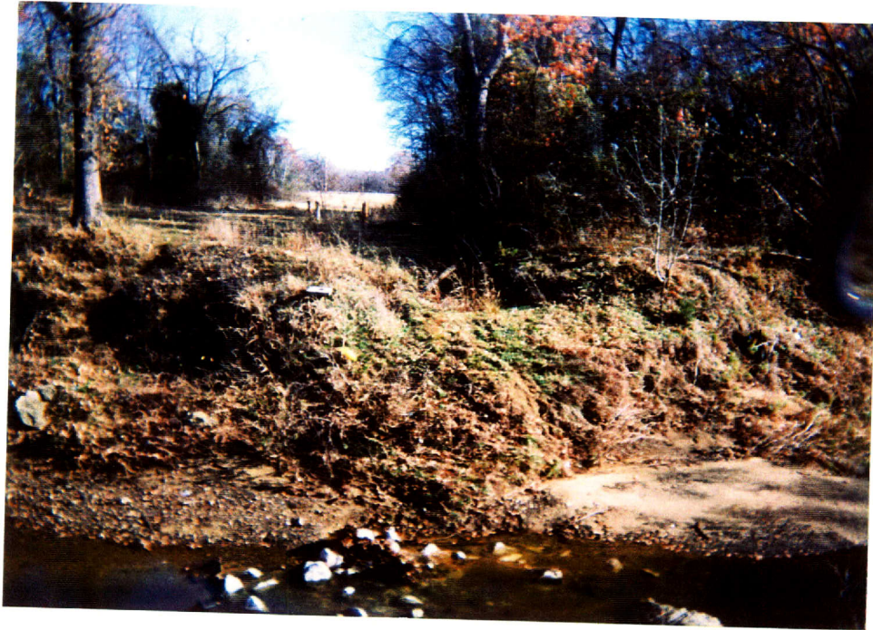
Figure 4. Gas pipeline extending above ground on the northeast bank of Timber Creek. An old pipe can be seen lying on the bank. Shovel test 9 was placed a meter away from creek channel in eastern portion of the picture adjacent to tree line.
