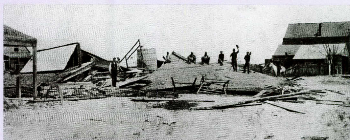
This store on East Main Street was completely demolished in the Indianola Storm of 1886.
