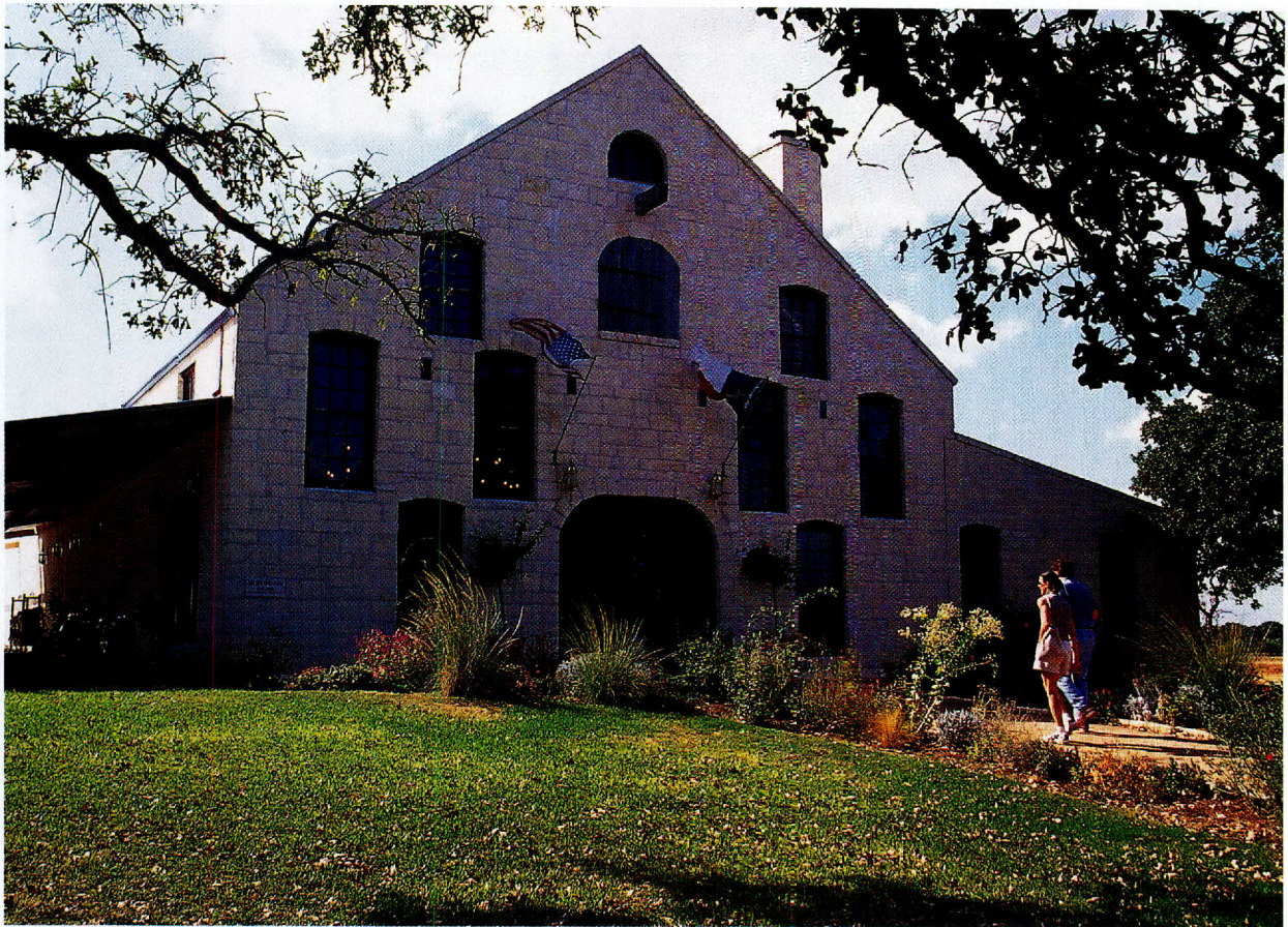
Built with local limestone, Becker Vineyards' winery and large tasting room resemble a German stone barn. Nearby, an 1890 log cabin serves as a rustic bed and breakfast.
