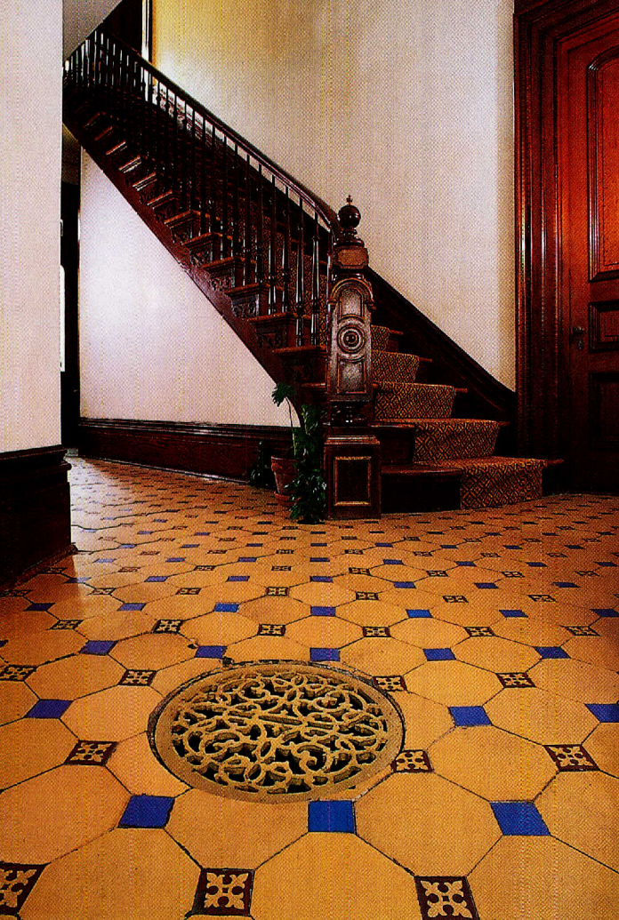
Showy English tile, original to the home, surrounds a cast-iron heat register in the vestibule.
