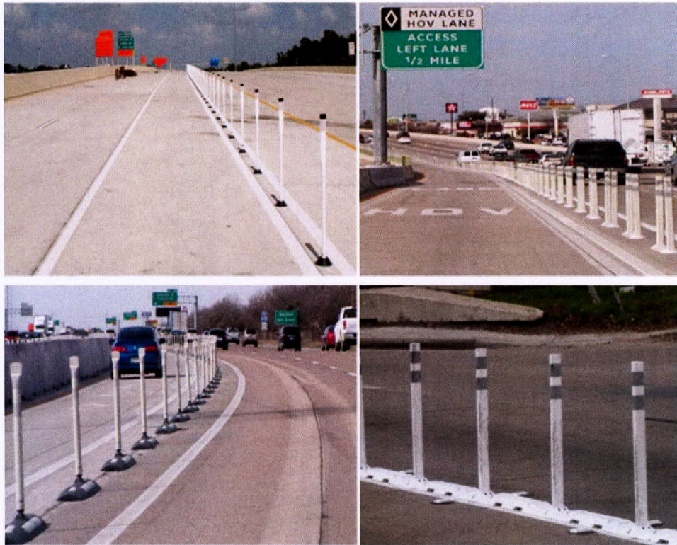
Figure 1. Examples of Pylon Devices.
