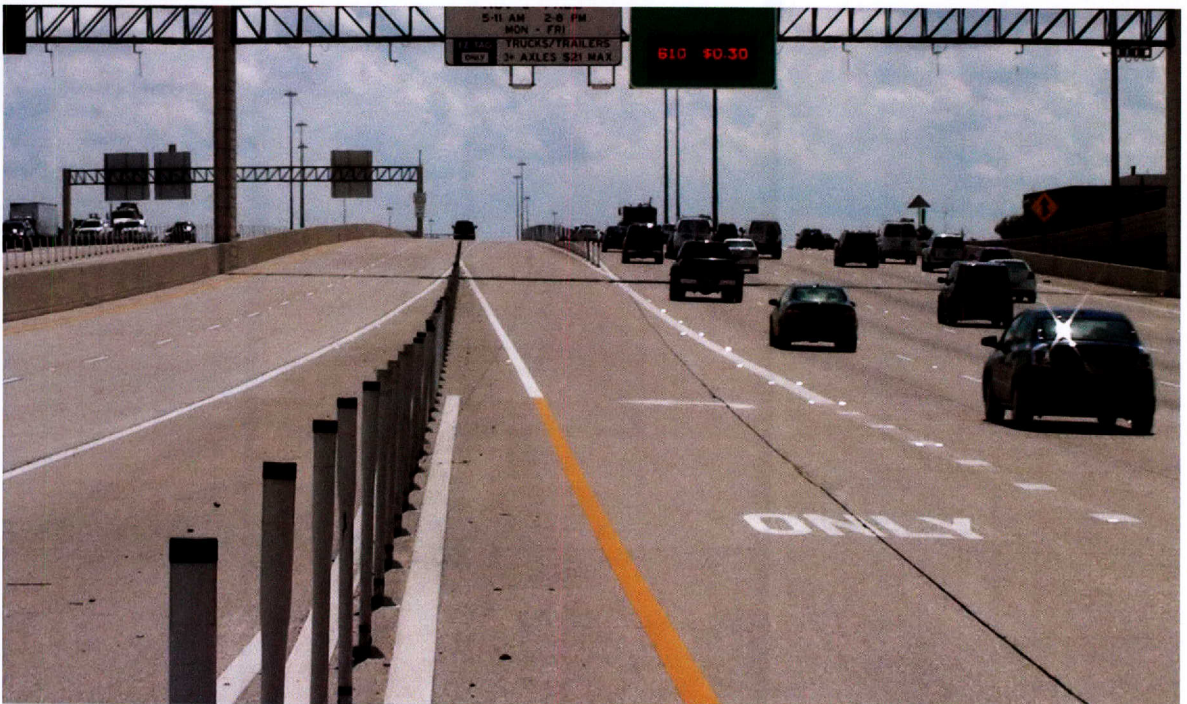
Figure F-4. Entrance to IH 10 EB Managed Lane at Bunker Hill Road.
