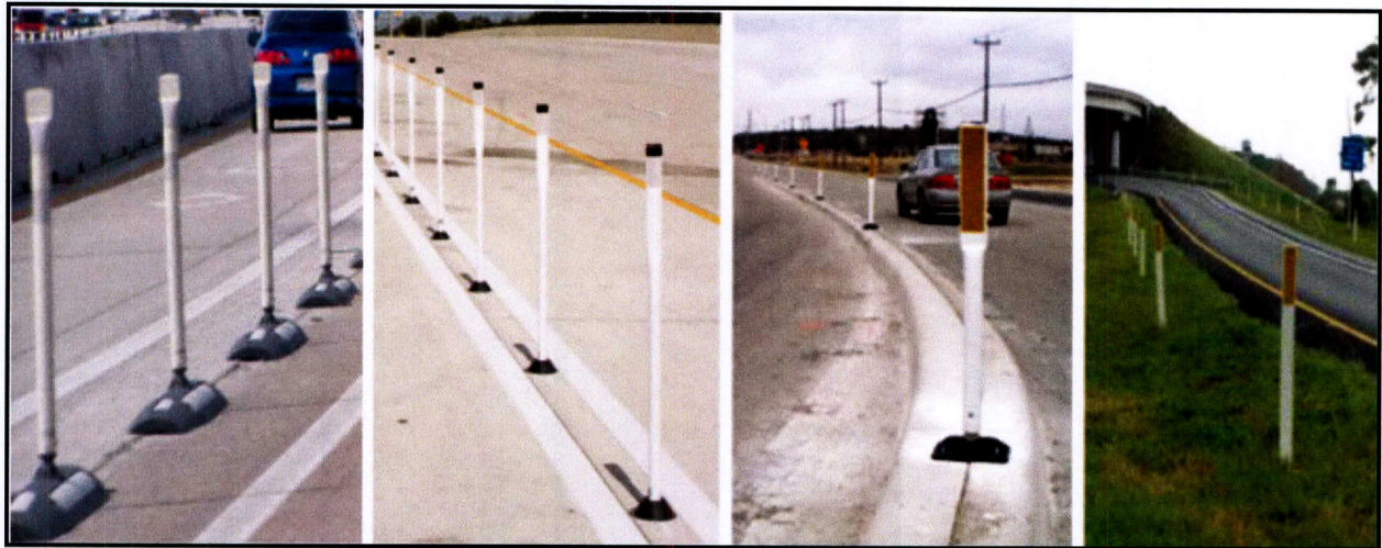
(a) Curb Mounted (b) Pavement Mounted (c) Surface Mounted (11) (d) Embedded (11)
