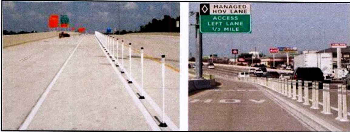
Figure 6. Pylon Implementation on IH 10 Katy Managed Lane (Houston) and US 75 HOV (Dallas) (6).
