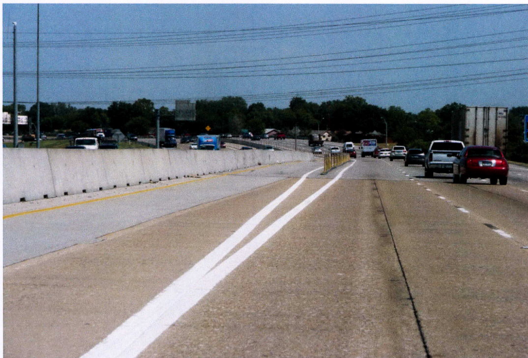
Figure F-2. Entrance to IH 635 NB HOV at Oates Drive (just North of IH 30).
