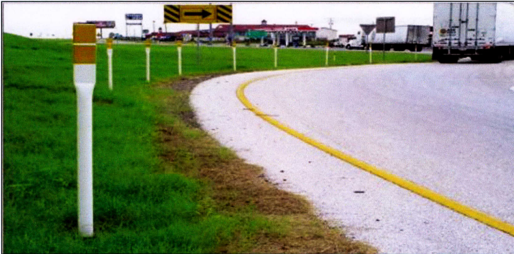
Figure 5. Example of Pylons Used for Curve Delineation (11).
