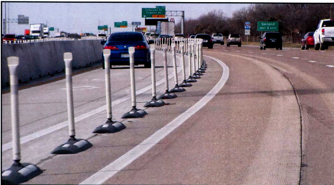
Figure 17. Curb-Pylon Implementation on IH 635 in Dallas (8).
