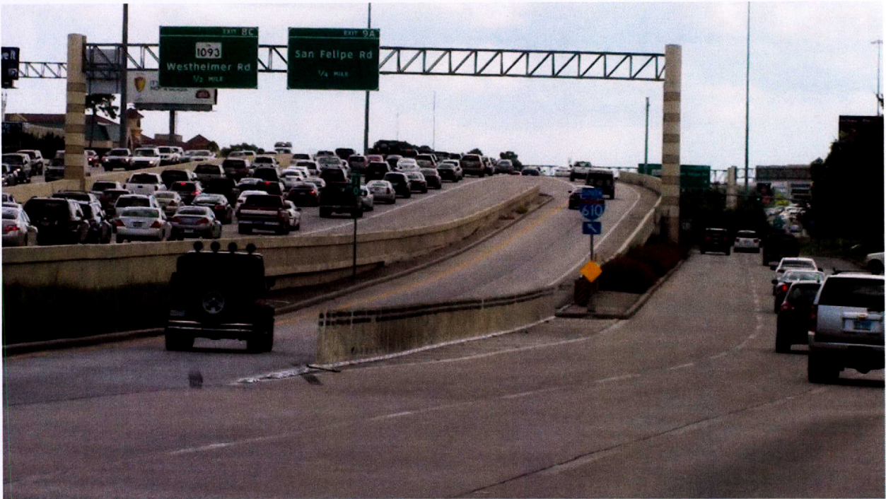
Figure F-13. IH 610 West Loop SB Woodway Drive Entrance Ramp in Houston, TX.
