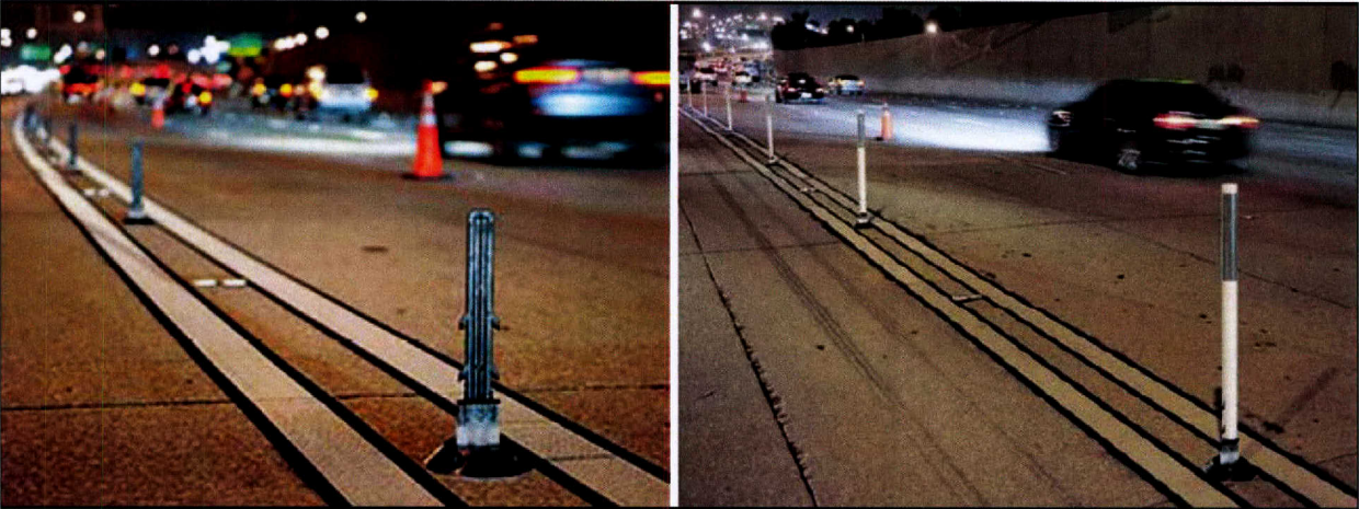
Figure 19. Pylons Used on IH 95 Express Lanes in Miami, Florida (6).
