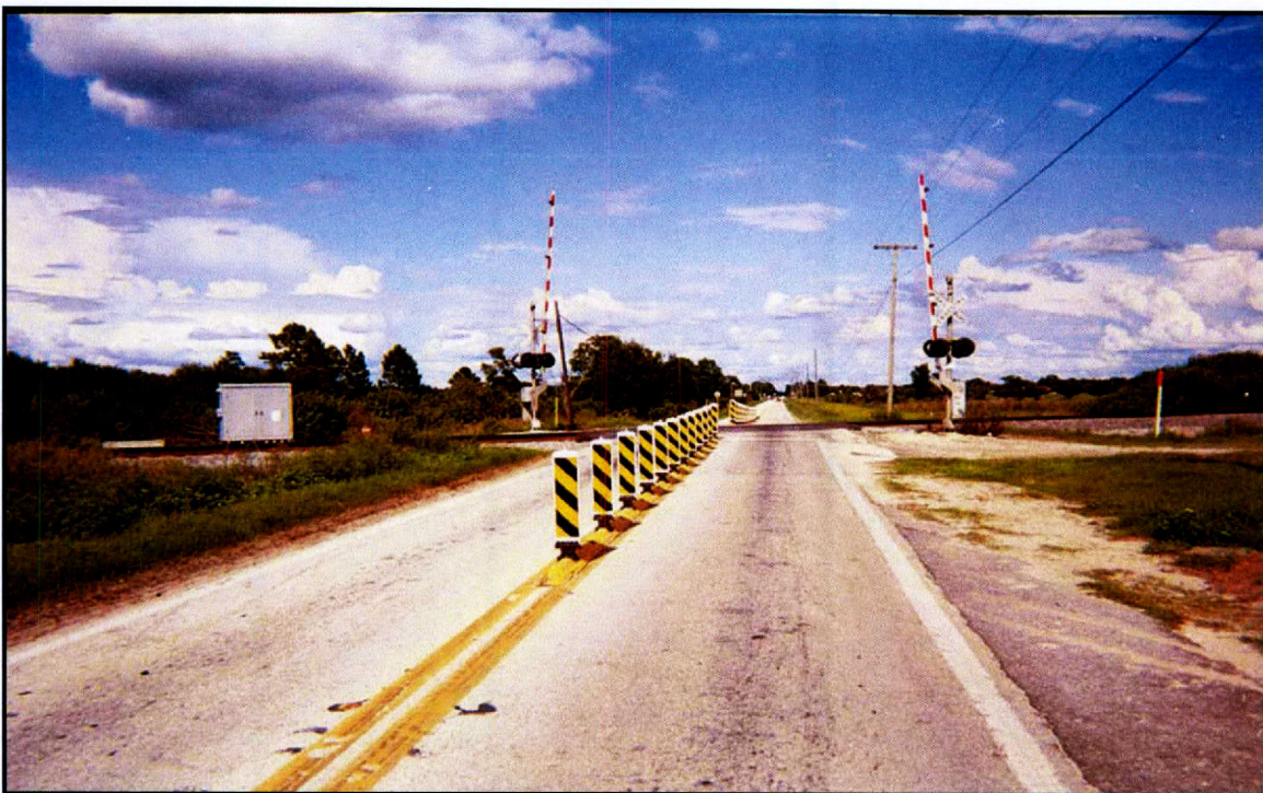
Figure 7. Example of Curb-Pylons Used at Highway-Rail Grade Crossing (4).
