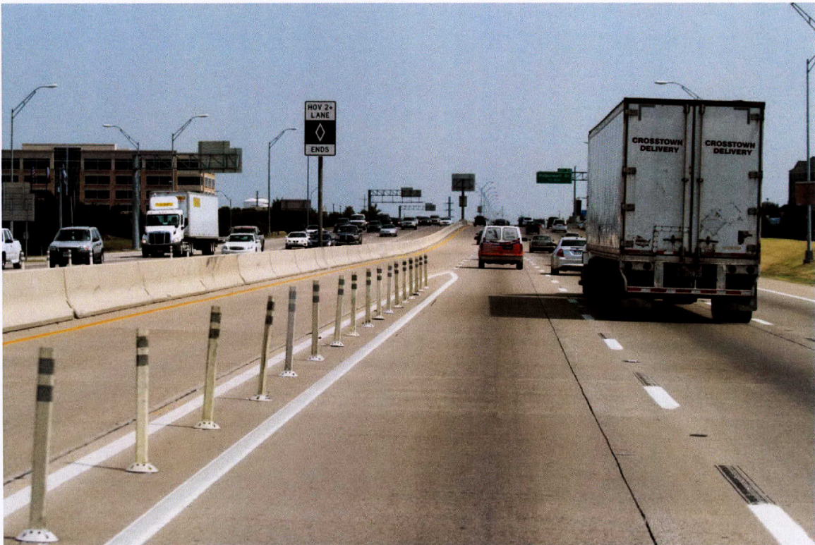
Figure F-6. Exit from US 75 NB HOV Lane at Bethany Drive (Dallas District).
