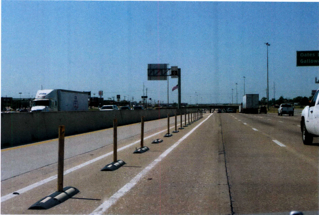
Figure F-7. Exit from IH 635 SB HOV Lane at Oates Drive (Dallas District).
