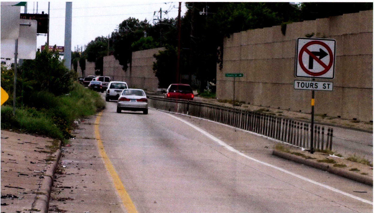
Figure F-16. US 59 WB Beechnut St Exit Ramp in Houston, TX.
