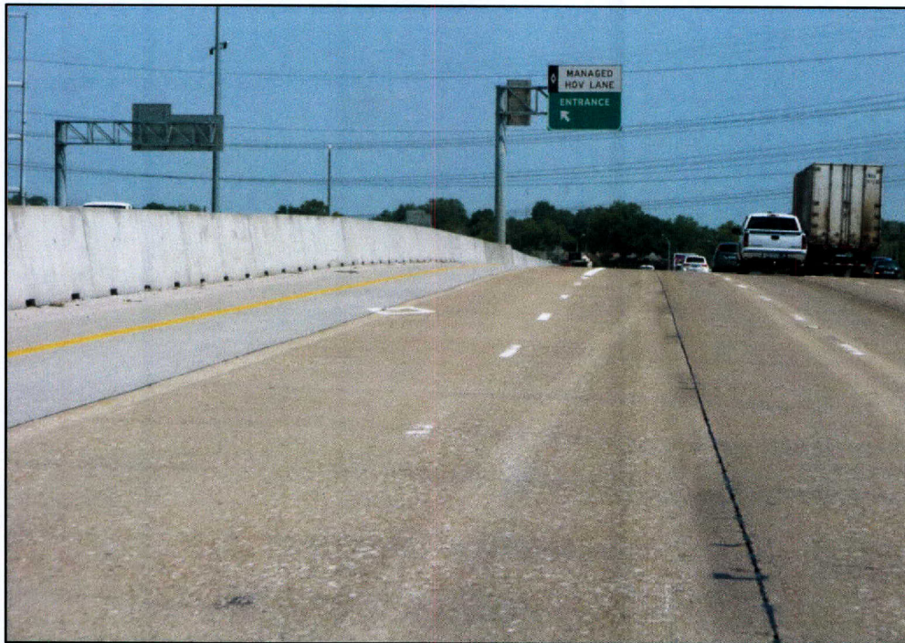
Figure 40. Vertical Curvature on Approach to the HOV Lane Entry at IH 635 Northbound at Oates Road Study Site, Mesquite, Texas.
