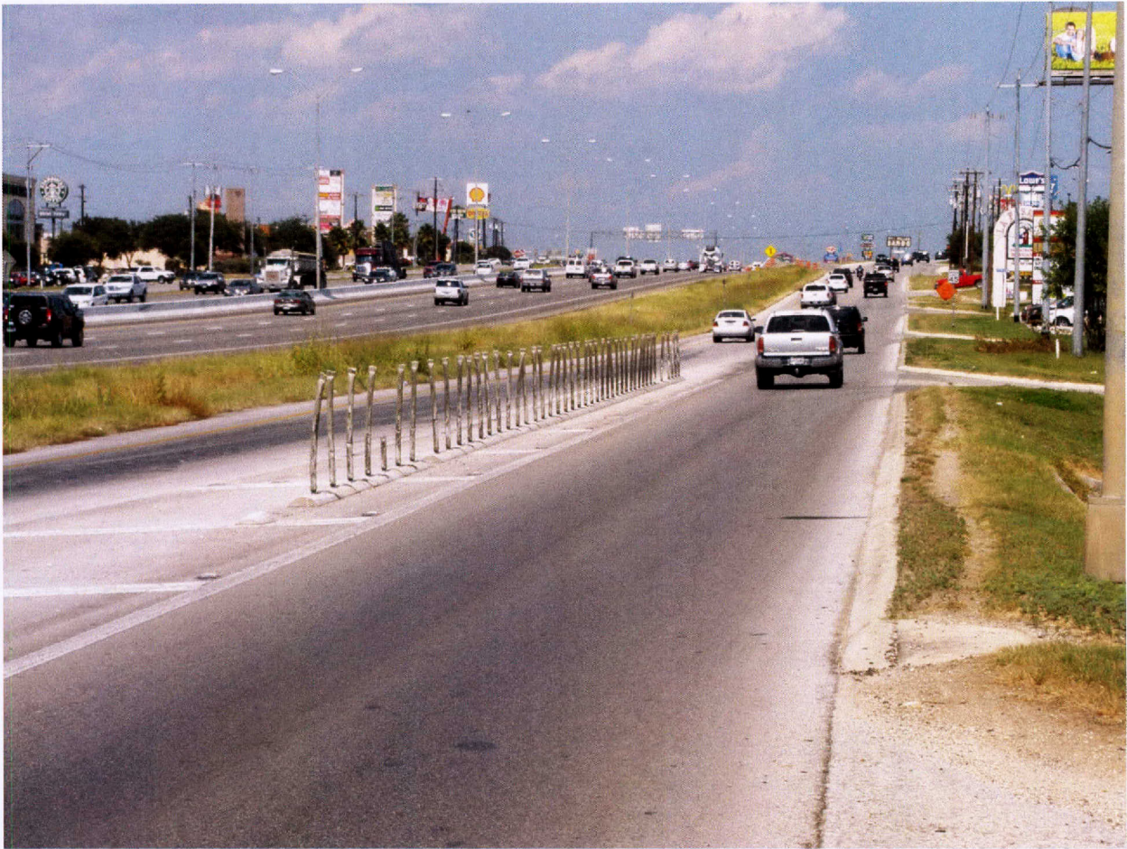
Figure F-17. IH 35 NB FM 3009 Exit Ramp in San Antonio, TX.
