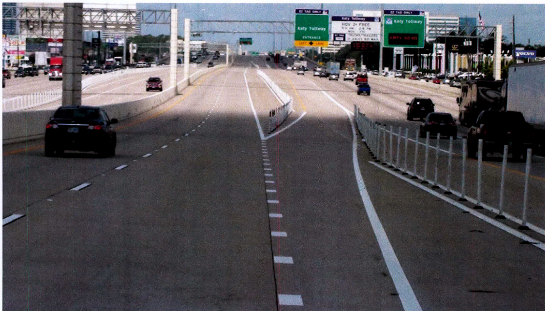
Figure F-8. Exit from IH 10 Katy Managed Lane at Tully Road (between Beltway 8 and SH 6 in Houston, TX).
