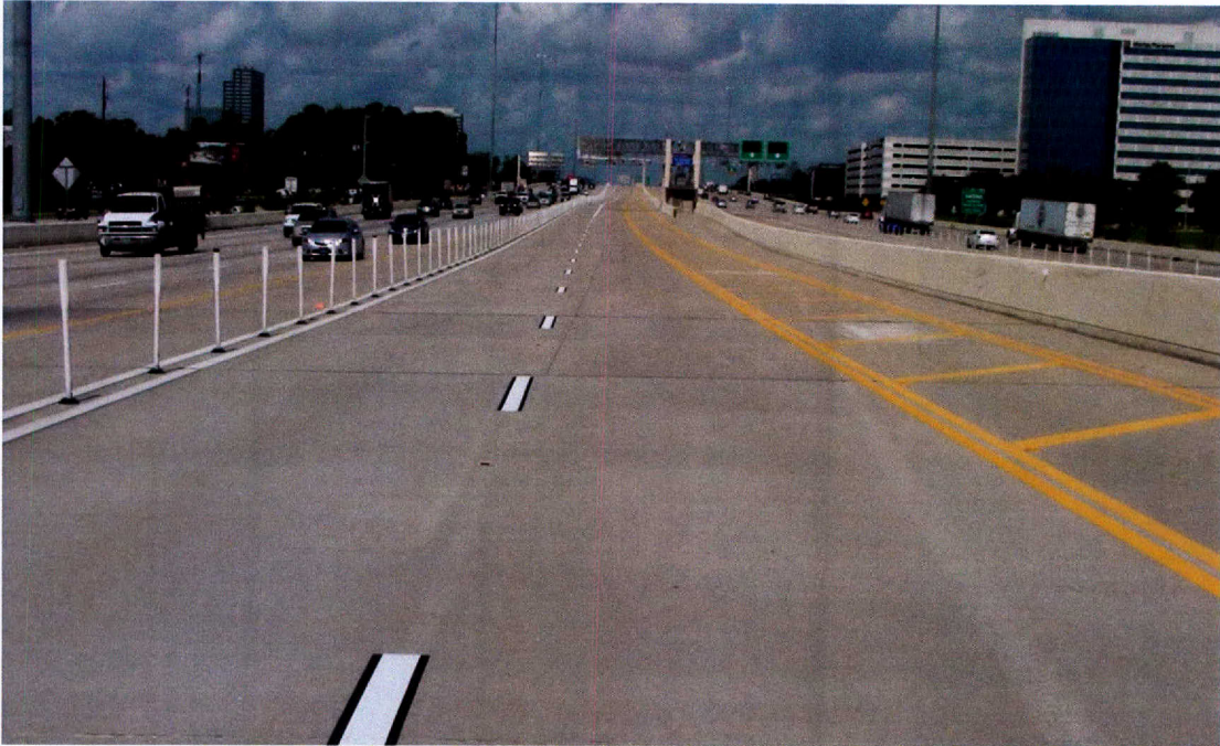
Figure F-11. IH 10 Katy Managed Lane EB near Dairy Ashford Road.
