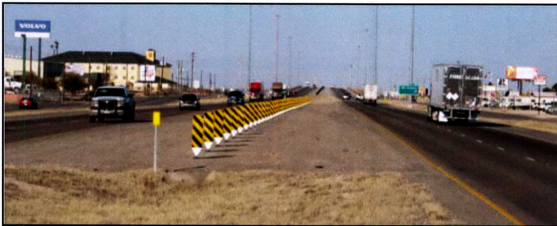
Figure 11. Use of Vertical Panels to Prevent Crossover Movements on IH 20, Odessa, Texas.
