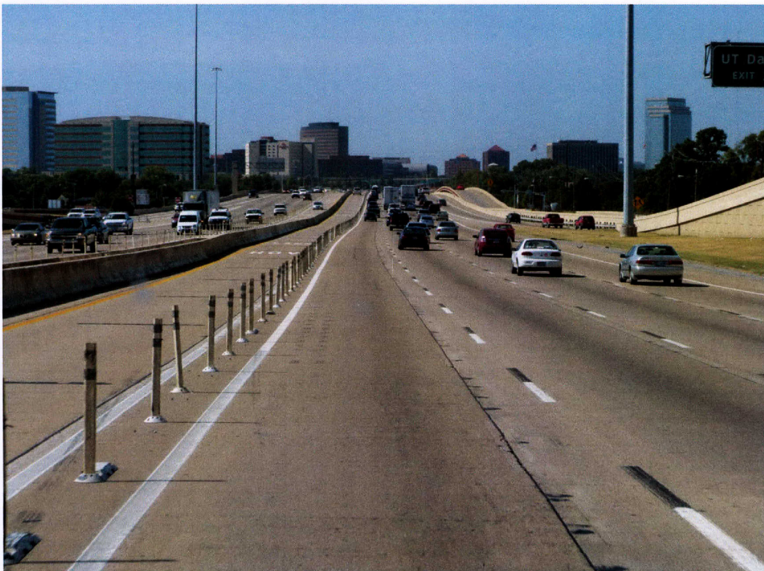
Figure F-10. US 75 SB HOV Lane South of George Bush Turnpike.
