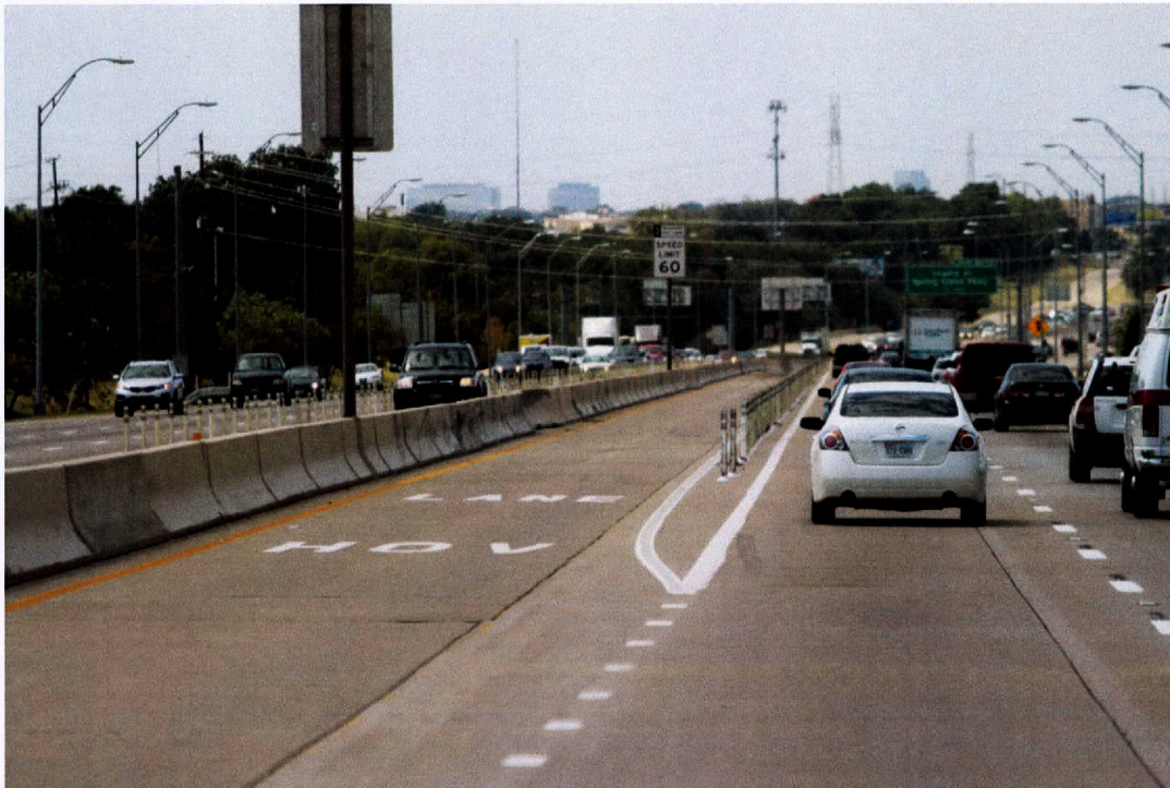
Figure F-1. Entrance to US 75 SB HOV at Bethany Drive.
