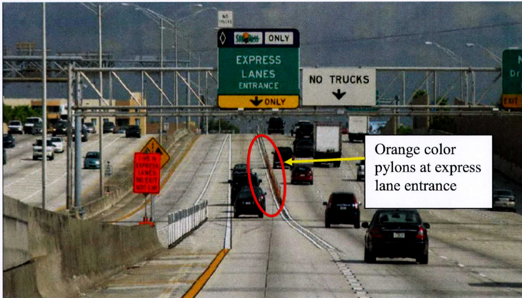
Figure 20. Orange Color Pylons Used to Increase Contrast at Access Points on IH 95 Express Lanes (6).
