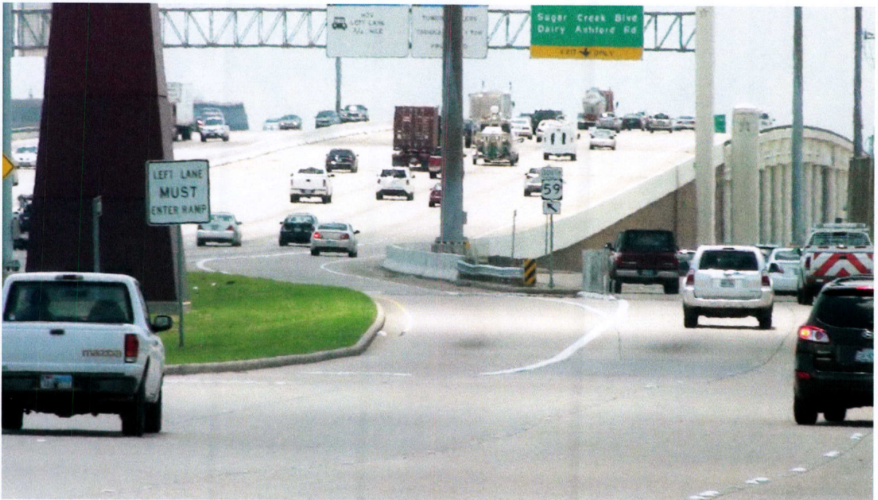
Figure F-15. US 59 WB Kirkwood Rd Entrance Ramp in Houston, TX.
