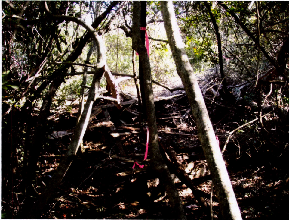
Figure 14. Site 41HR1131 Boudreaux Farm collapsed building, facing east.
