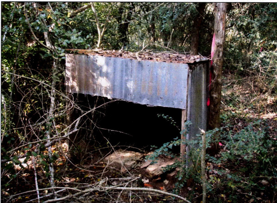
Figure 15. Site 41HR1131 Boudreaux Farm well shed, facing northwest.
