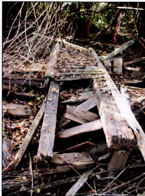
Figure B-10. 41HR1131 Boudreaux Farm bulldozed east wall, facing west.
