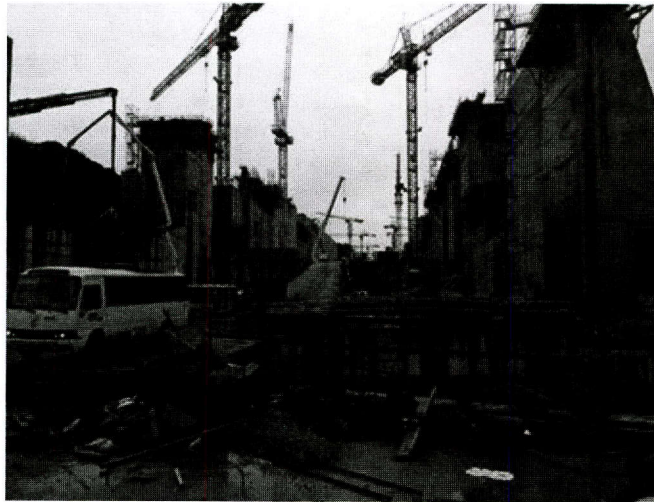
Figure 3 PCE under construction
