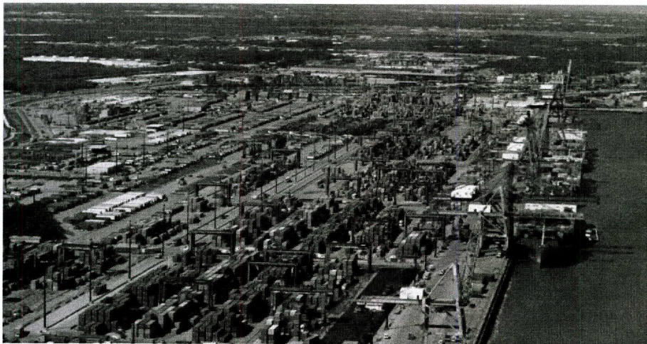
Figure 9 Barbours Cut Container Terminal
