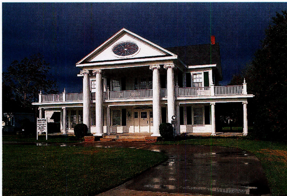
White Haven, originally built as a New England Colonial-style mansion in 1915, was transformed into the Southern Greek Revival style when the second owners added large verandas and columns. Today, the home welcomes guests with Victorian-era furniture, a screen that belonged to Empress Carlota of Mexico, and candelabras that once provided light for the Shah of Persia.
