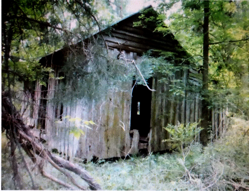
Figure 22. North side of house at 41RK196, facing southwest.
