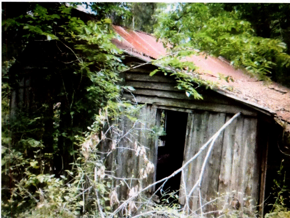
Figure 25. North side of house at 41RK196, facing south-southeast.
