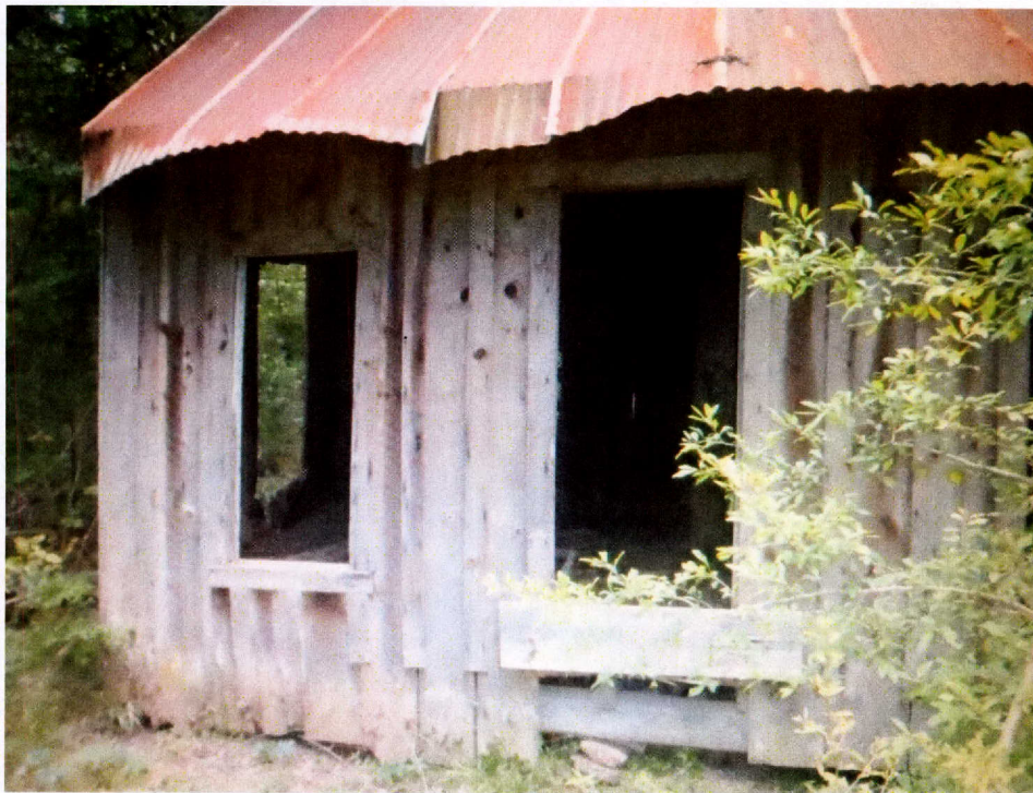
Figure 23. East side of house at 41RK196, facing west.
