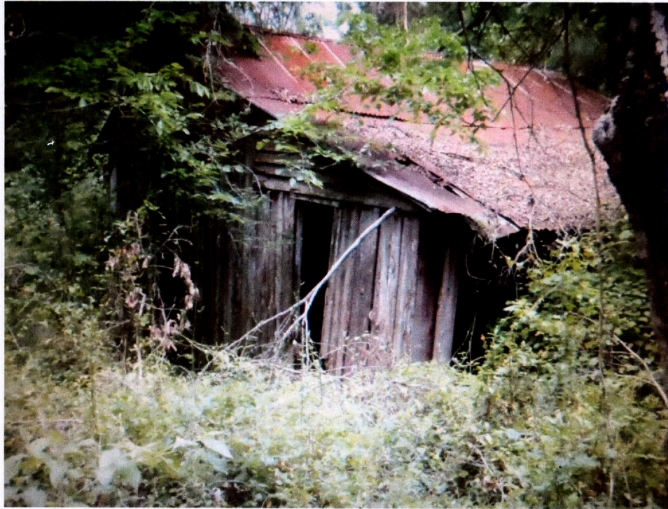
Figure 24. Northwest corner of house at 41RK196, facing southeast.
