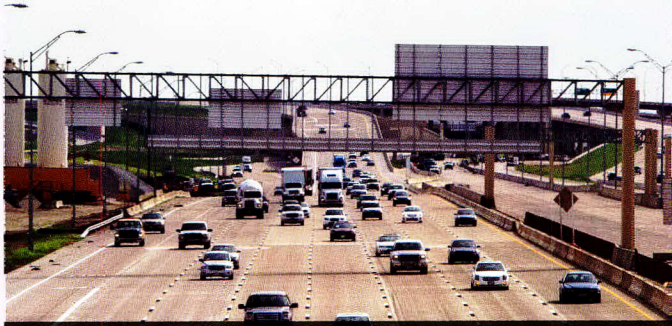
The project, TxDOT's first public-private partnership to open in North Texas, doubles the capacity of the existing highway from 12 to 24 lanes.
