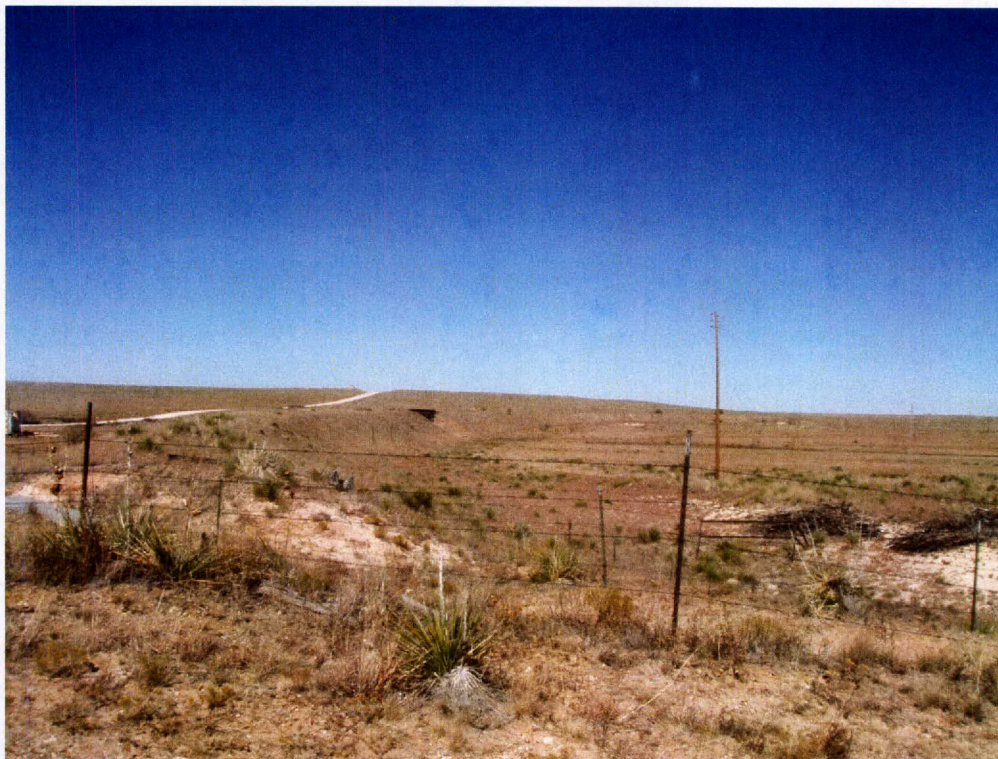
b) Bridge Crossing Cottonwood Creek
