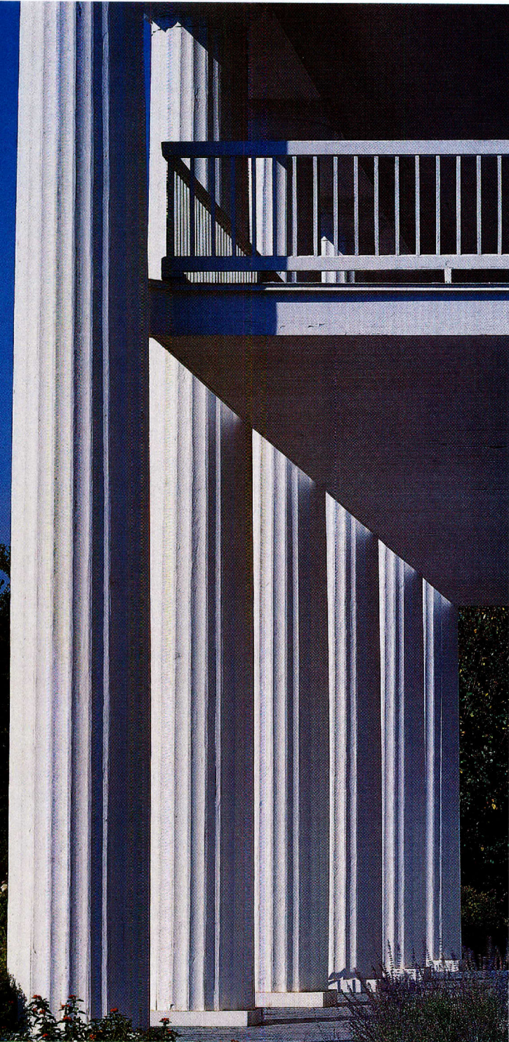
The tall front windows of the Earle-Harrison House open onto the porch. A common feature in antebellum mansions, the opened windows proved especially accommodating for the broad hoop skirts worn by women of the period.
