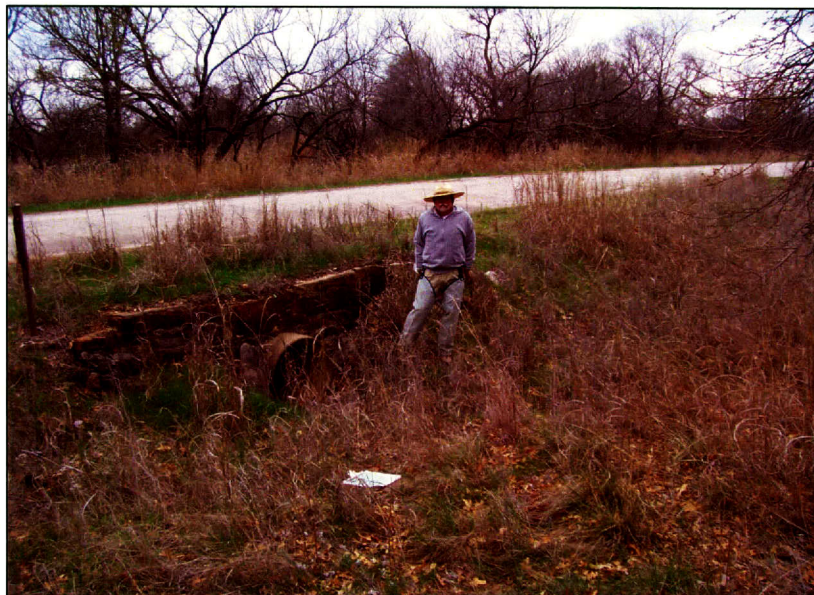
Figure 4. Lance Trask standing next to the culvert and culvert wall on the north of the concrete park road that marks the southern boundary of the pad site. View is to the southwest.
