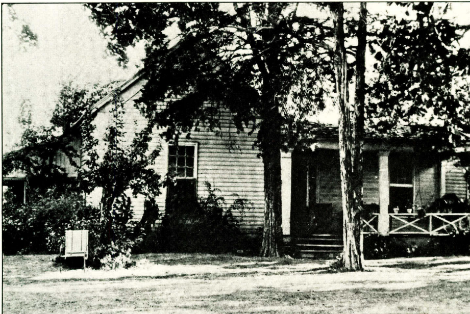
The original home of J. L. and Fannie P. Gilbert, founders of the Gilbert/Elliott Farm in Hopkins County, is seen as it stood in 1925. Still standing, the house was built after the Heritage farm was established in 1883.
