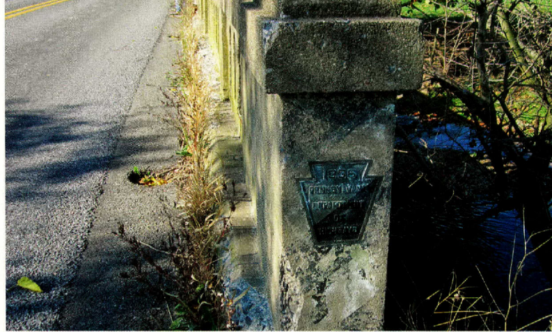
This Pennsylvania bridge rail is similar to thousands of others across the state. TTI has designed several bridge rail retrofit options the state is considering for implementation.
