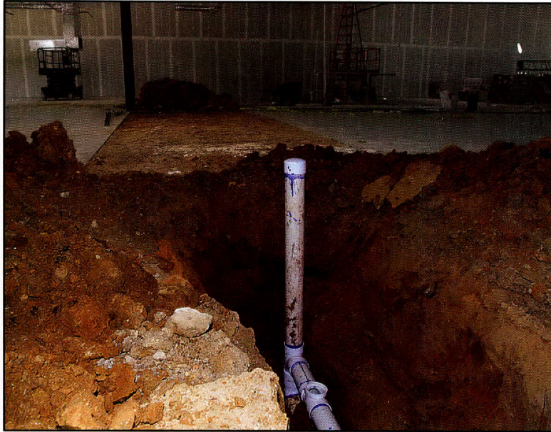
"LEAVE OUTS" IN FOUNDATIONS at Corporate Centre Kirby accommodate the added plumbing medical offices need.
