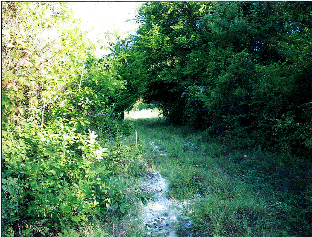
Figure 4. The proposed pipeline route will be placed in the center of the dirt two-track road which is covered with asphalt chunks and gravel. Note stake marking pipeline route. View is to the northwest.
