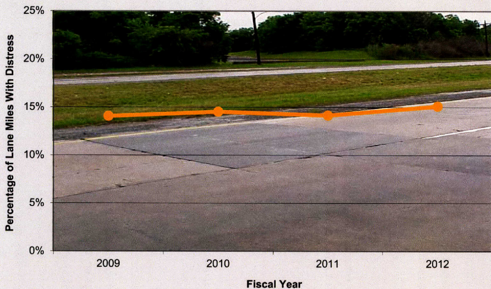
CRCP Concrete Patches (rated), FY 2009-2012
