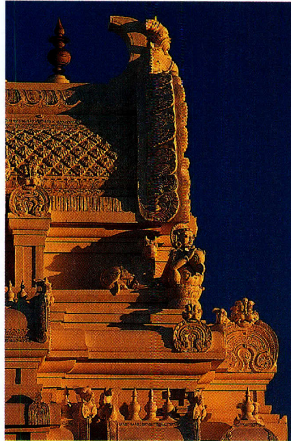
Once made from stone, detailed tower ornate- mentations like these are now created with concrete using special molds made by the temple artisans.
