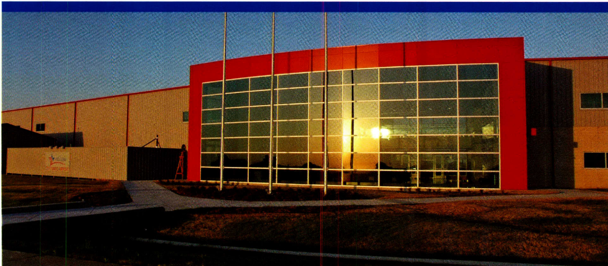
New terminal building at Texas State Technical College-Waco Airport in Waco, Texas
