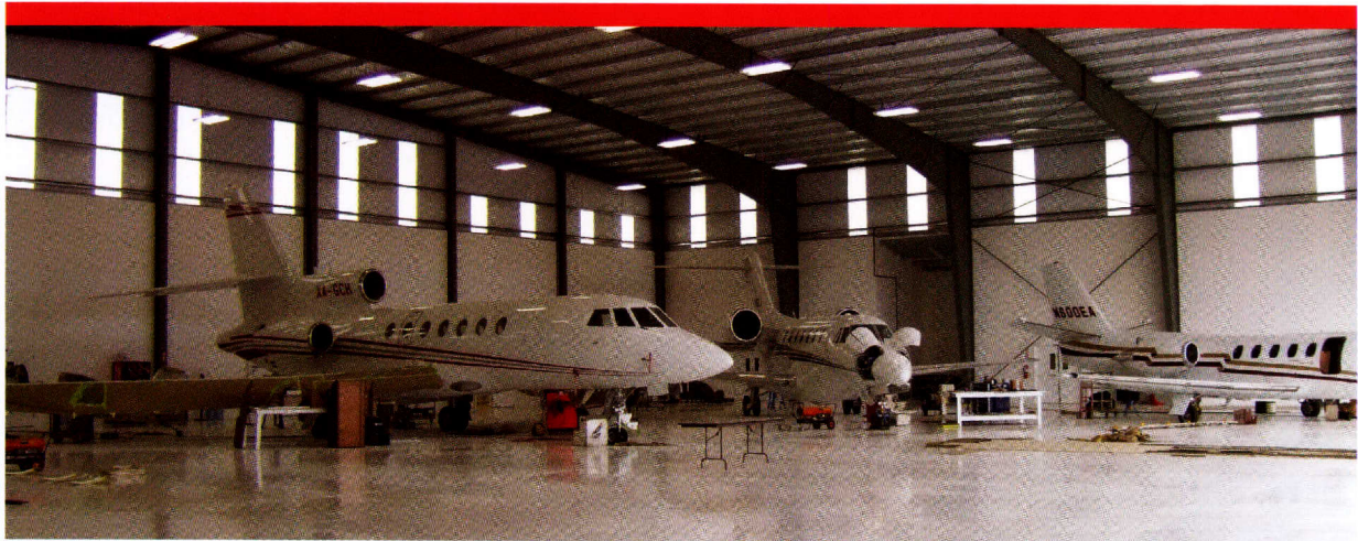
Airplane hangar in Uvalde, Texas
