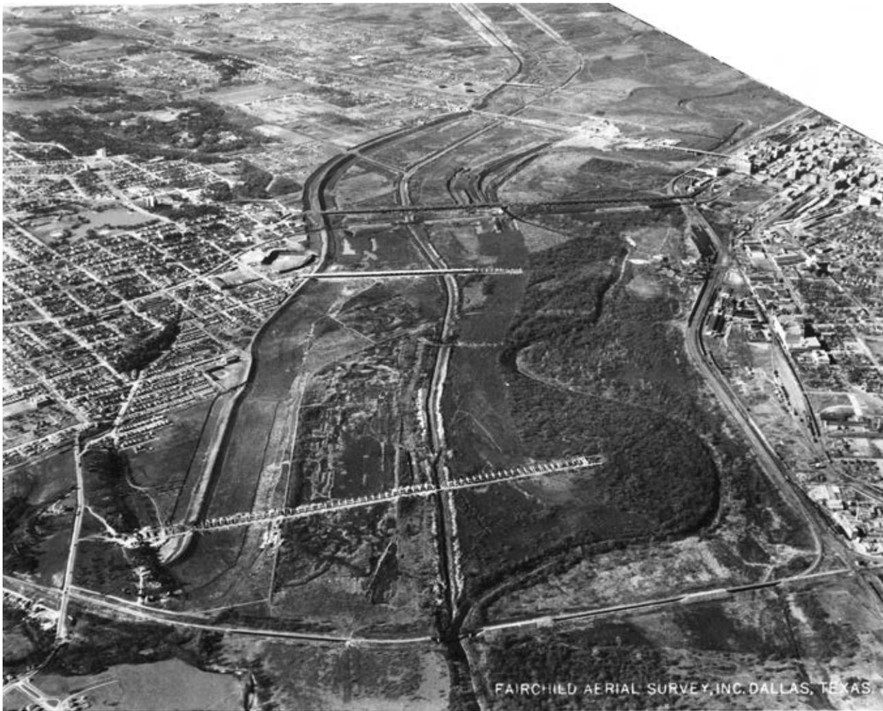
**This aerial photograph shows the newly constructed levees shortly before the Trinity River was diverted between them from its original, serpentine channel.**
