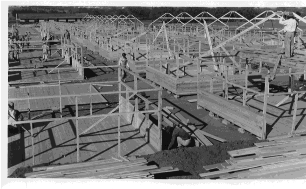
Constructing hutments, Camp Bowie, Texas
