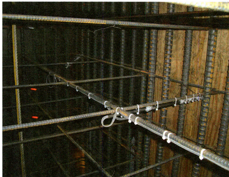
Figure 5.16: WBSB 9 Completed Instrumentation
