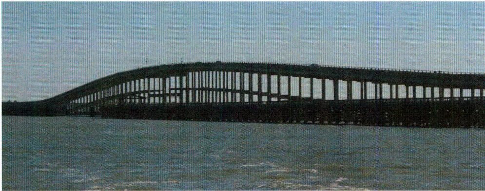
Figure 6.1: Copano Bay Bridge (Looking Northeast)
