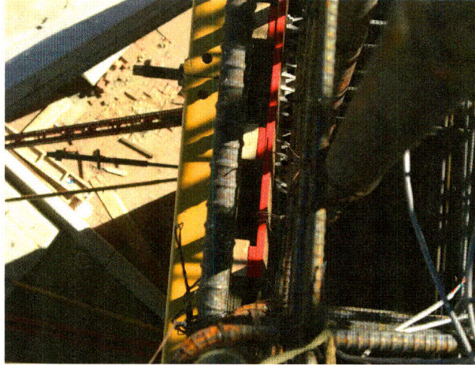
Figure 5.11: WBSB 9 Inset Formwork
